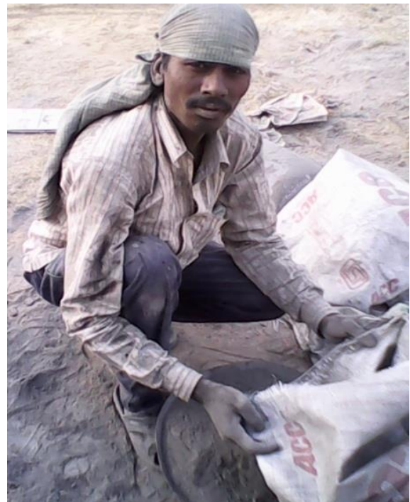
Figure 3: A worker without safety precaution
