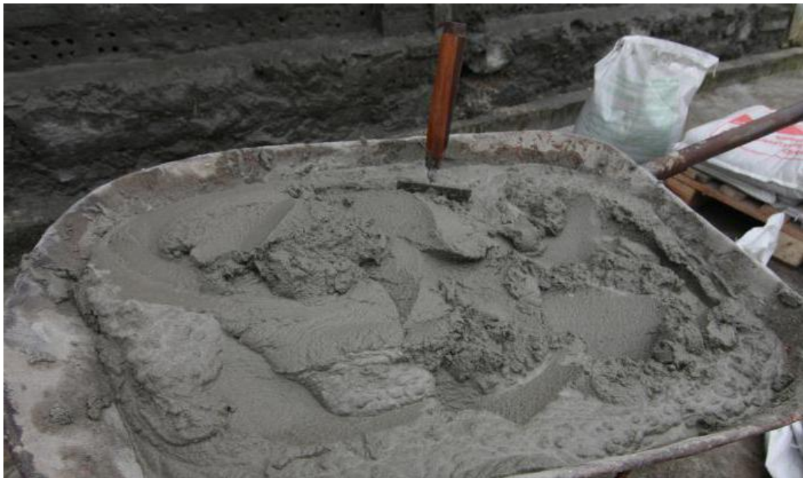
Fig 4: Cement Mortar [F4]
