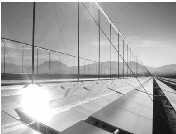
Figure 2.30. PE-1 1.4 MW powerplant [12].
