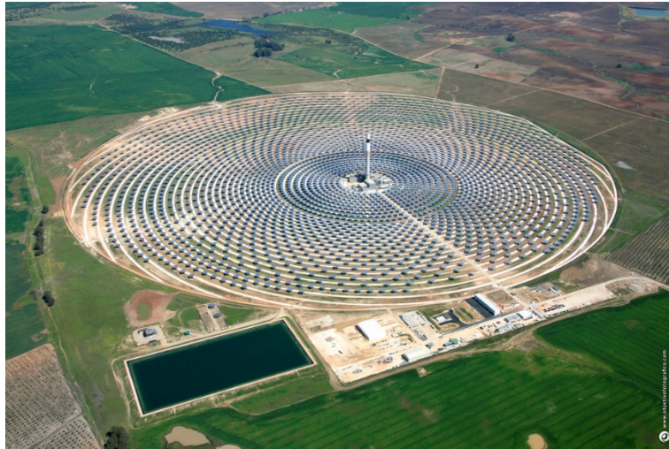
Figure 1.2. Central receiver tower plant Gemasolar plant [5].
