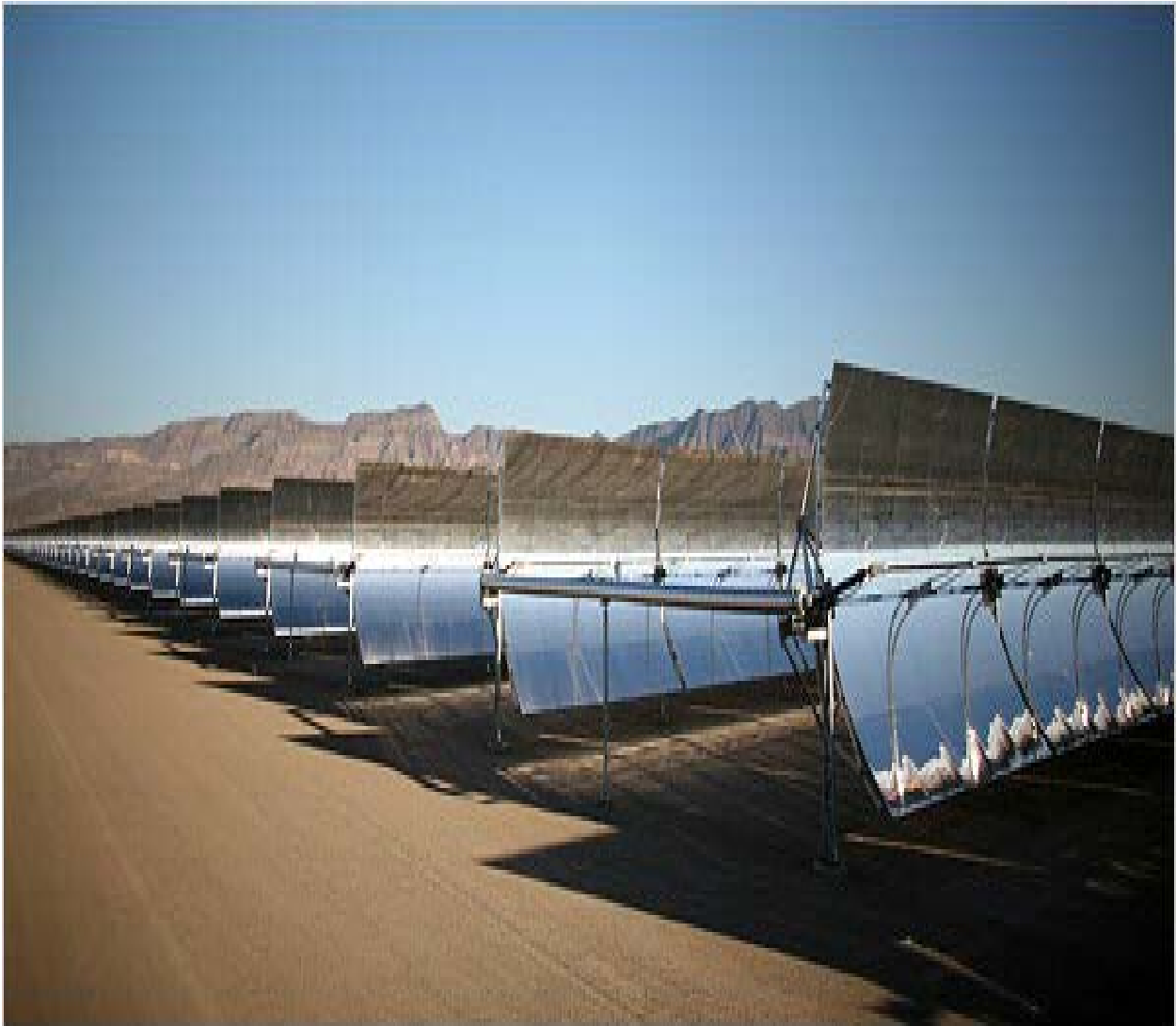
Figure 1.1. Parabolic trough collector Nevada Solar 1 [4].
