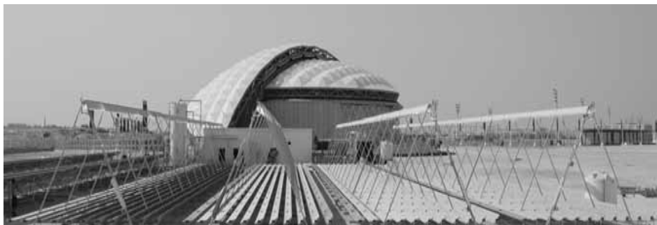
Figure 2.25. Industrial Solar Fresnel collector field in Doha absorption chiller [12].
