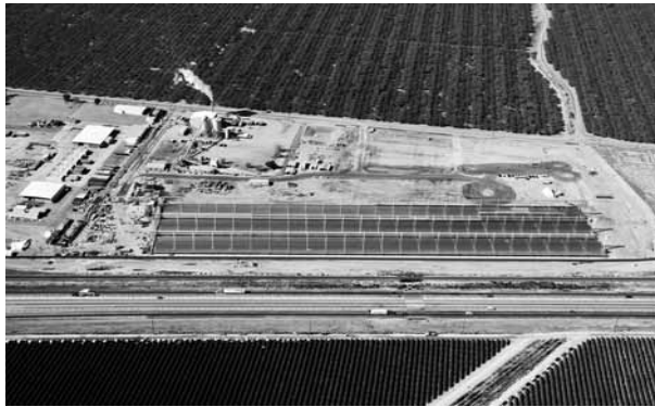
Figure 2.21. The three-line Kimberlina array [53].
