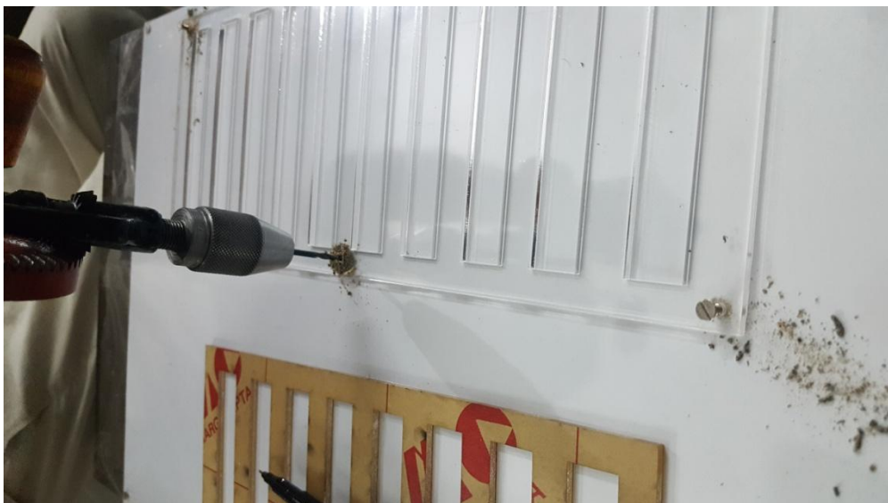
Figure 103 tightening the polycarbonate sheet
