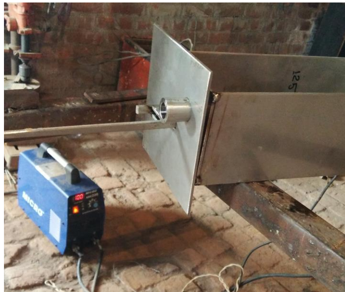
Figure 10 Fabrication of Internal Chamber (2)
