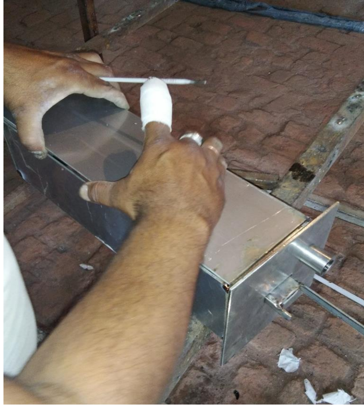
Figure 11 Fabrication of Internal Chamber (3)
