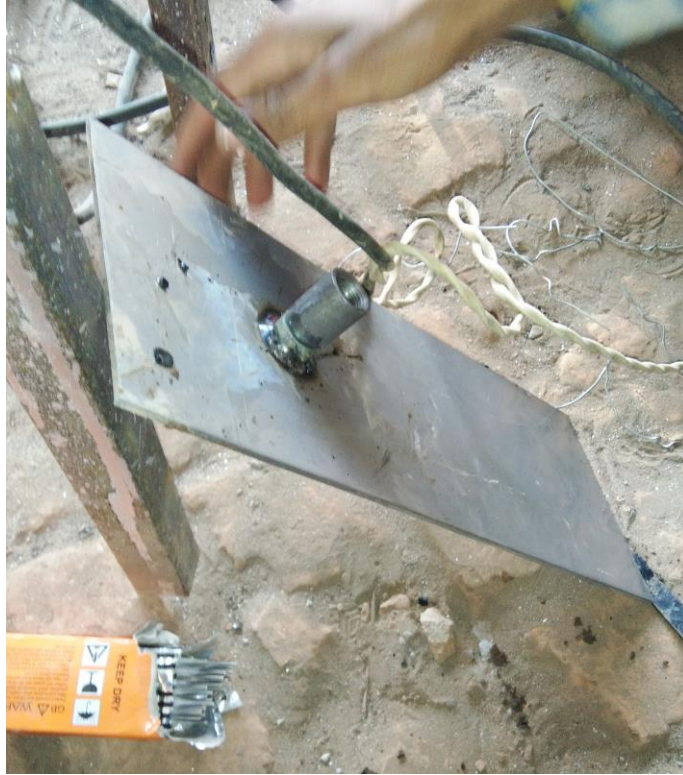
Figure 14 Fabrication of suction pump attachment accessory in external Chamber
