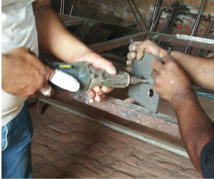
Figure 7 Preperation of specimen pockets and LN 2 inlet hole.
