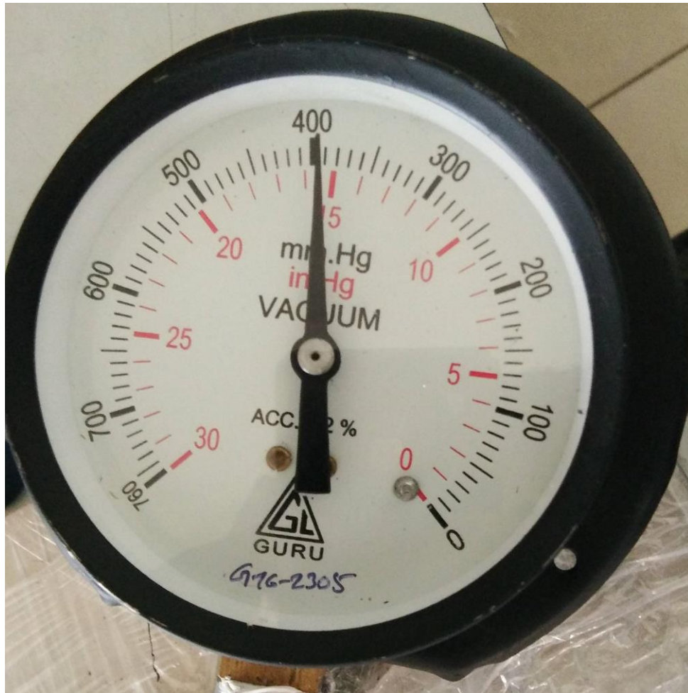
Figure 21 vacuum pressure reading after 30 minutes.
