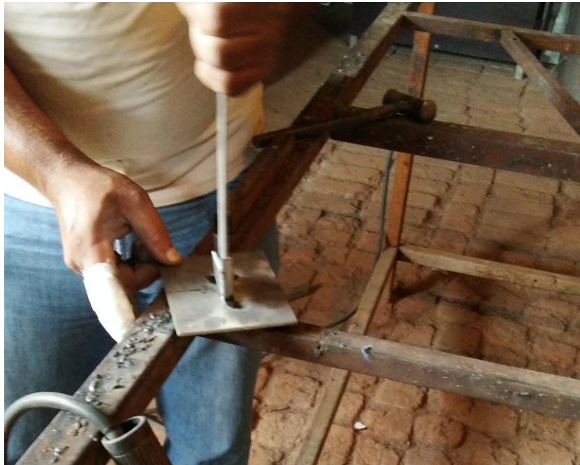
Figure 8 Preperation of Pocket for specimen.
