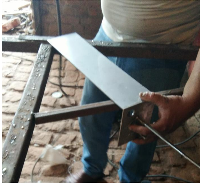
Figure 9 Fabrication of Internal Chamber (1)
