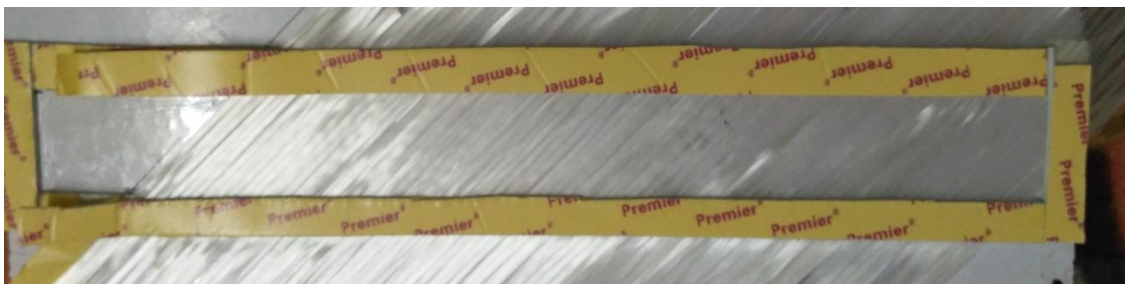
Figure 14 Placing the second layer of double tape
