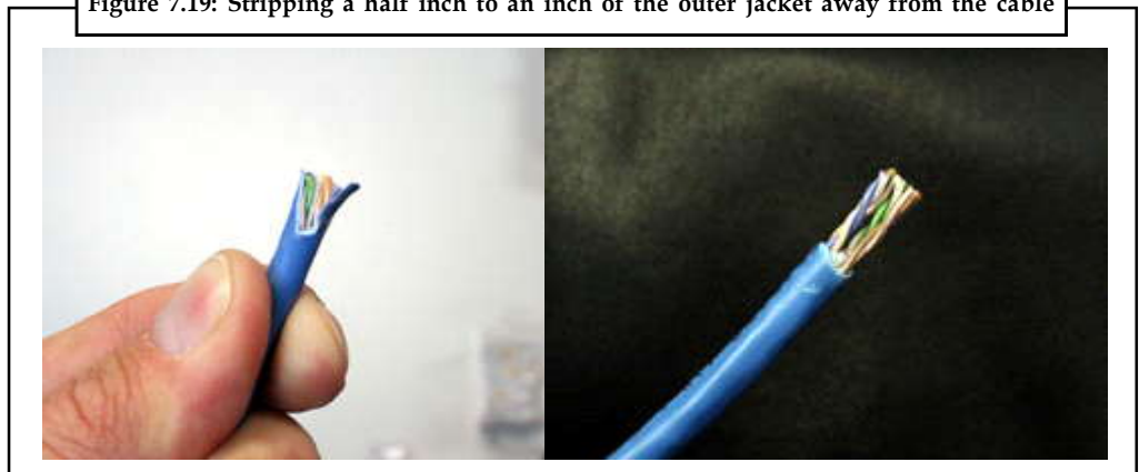
Figure 7.19: Stripping a half inch to an inch of the outer jacket away from the cable
