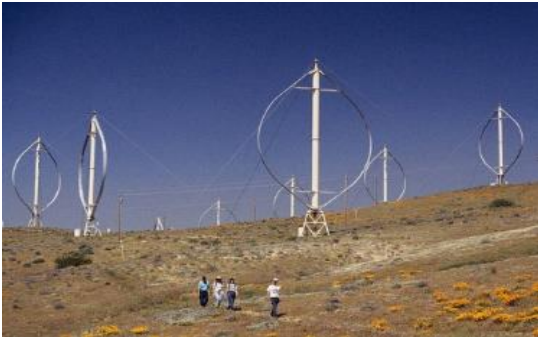
Figure 4.9: Site view of VAWT.
