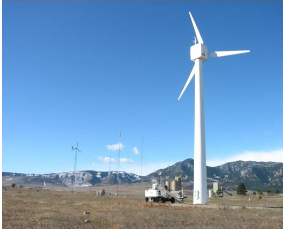
Figure.1.2 100-kW wind turbine.
