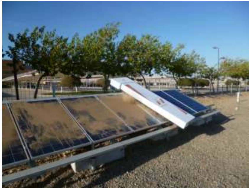
Figure5. NOMADD (NO-water Mechanical Automated Dusting Device)
