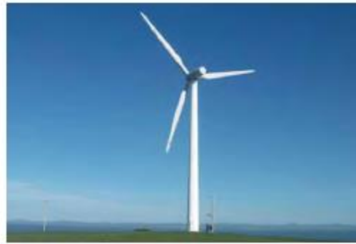
Figure 4 A standards WTG with 3 blades and horizontal axis
