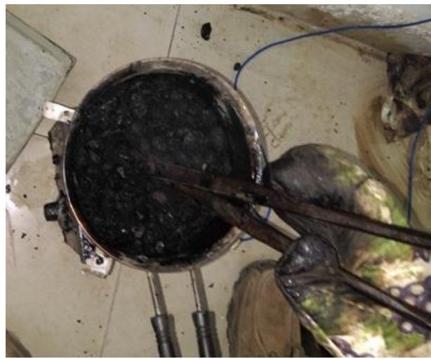
Figure No. 3.10 Mixing of aggregates and binder
