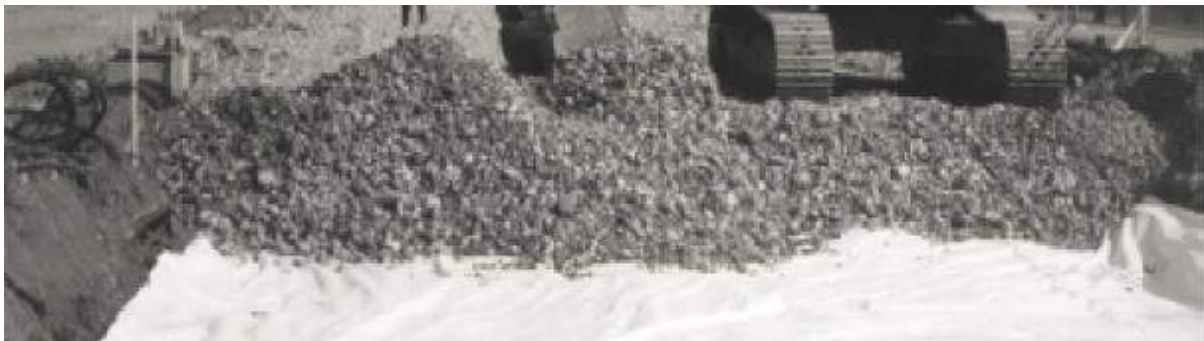
Fig3: Granular base course material
