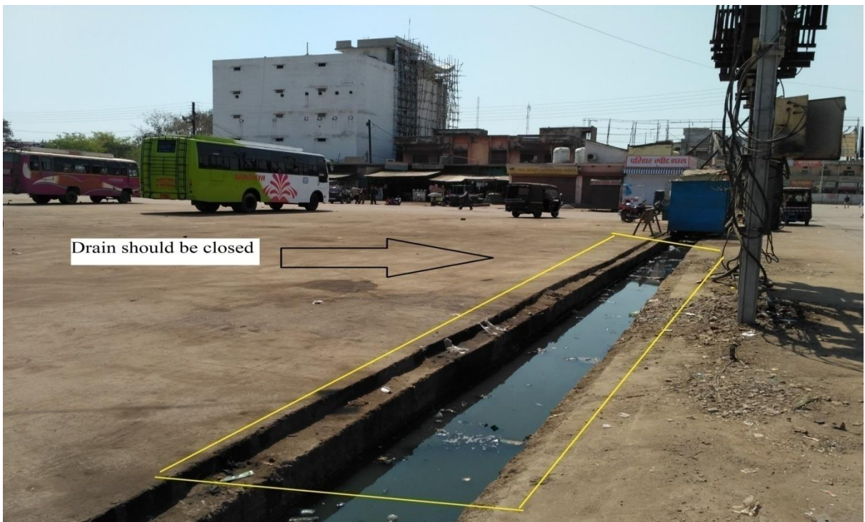
Fig-4.5 Open drains
