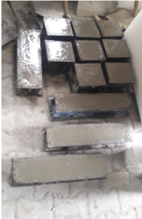
Fig. 4: Casting of moulds
