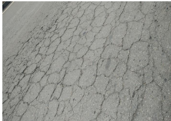
Fig.28: Alligator cracks at the existing pavement at Khashi Nagar
