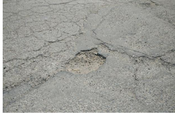
Fig.35: Alligator cracking and Depression at near Chachoki. Fig.36: Depression at Chauckoki Village.
