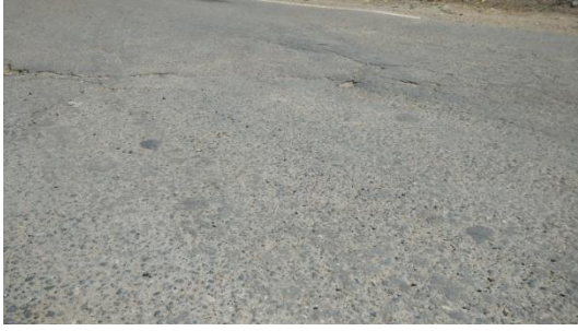
Fig.19: Polished Aggregate of Existing
