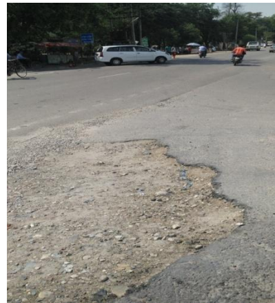
Fig.8: Patches and Alligator cracks near Hanuman Mandir Fig.9: Edge cracks on light wala chowk.
