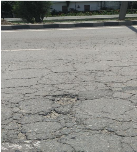
Fig.25: Potholes and alligator cracks near Haddi meal. Fig.26: a big patch near Saprur.
