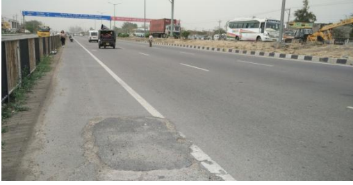
Fig.18: Patching of road near civil hospital. pavement.
