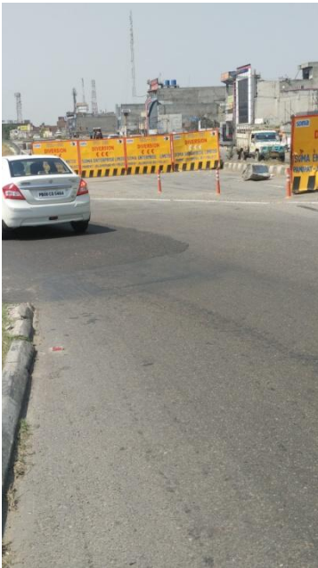
Fig.12: Patch near rail bypass
