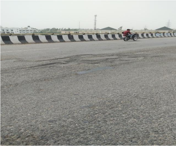
Fig.20: Failures on the over bridge at kashi Nagar chandighar bypass.
