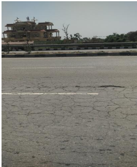
Fig.27: Alligator cracking at KASHI Nagar
