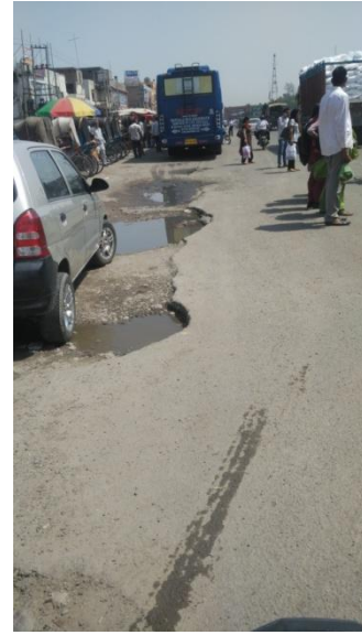
Fig.6 :Cracks and bleeding on the road near GTC Meal area. Fig.7: Edge cracking near bus stand
