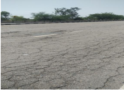
Fig.35: Alligator cracking and Depression at near Chachoki. Fig.36: Depression at Chauckoki Village.
