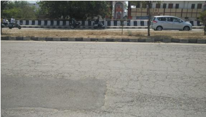
Fig.8: Patches and Alligator cracks near Hanuman Mandir Fig.9: Edge cracks on light wala chowk.
