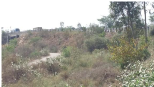
Fig.38: Haddi over bridge
