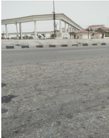
Fig.22: Existing pavement of Alligator and Depression near Cabana resort
