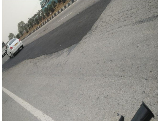
Fig.25: Potholes and alligator cracks near Haddi meal. Fig.26: a big patch near Saprur.
