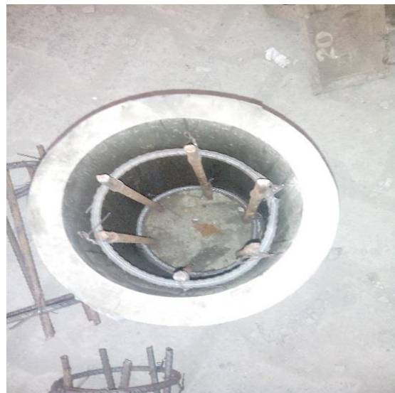
Fig. no.3: Arrangement of steel rebars within frame work.
