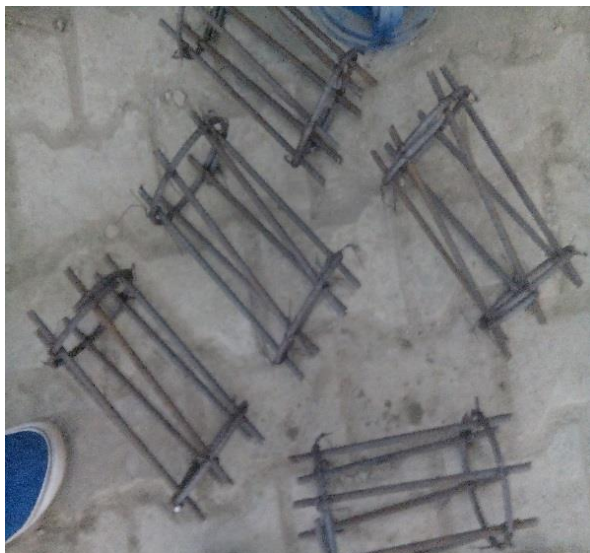
Fig. no.3: Arrangement of steel rebars within frame work.
