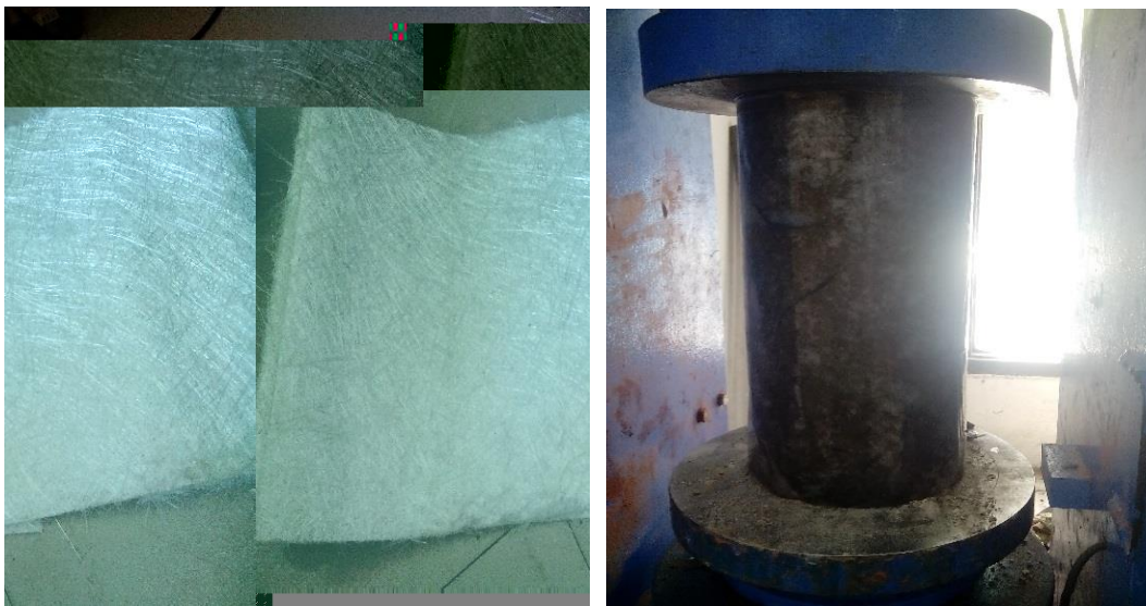
Fig. 4: Glass fiber and the column wrapped with GFRP.
