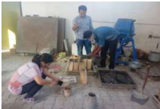
Figure 6.13 casting of columns
