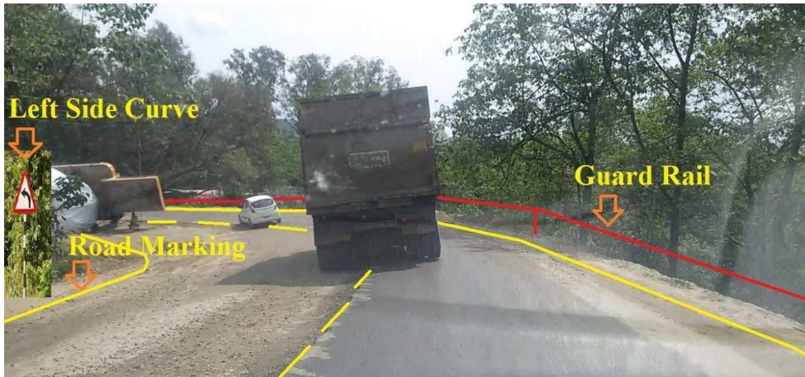
Fig 4.4: Suggestions for improvement for Mubarakpur accident spot.
