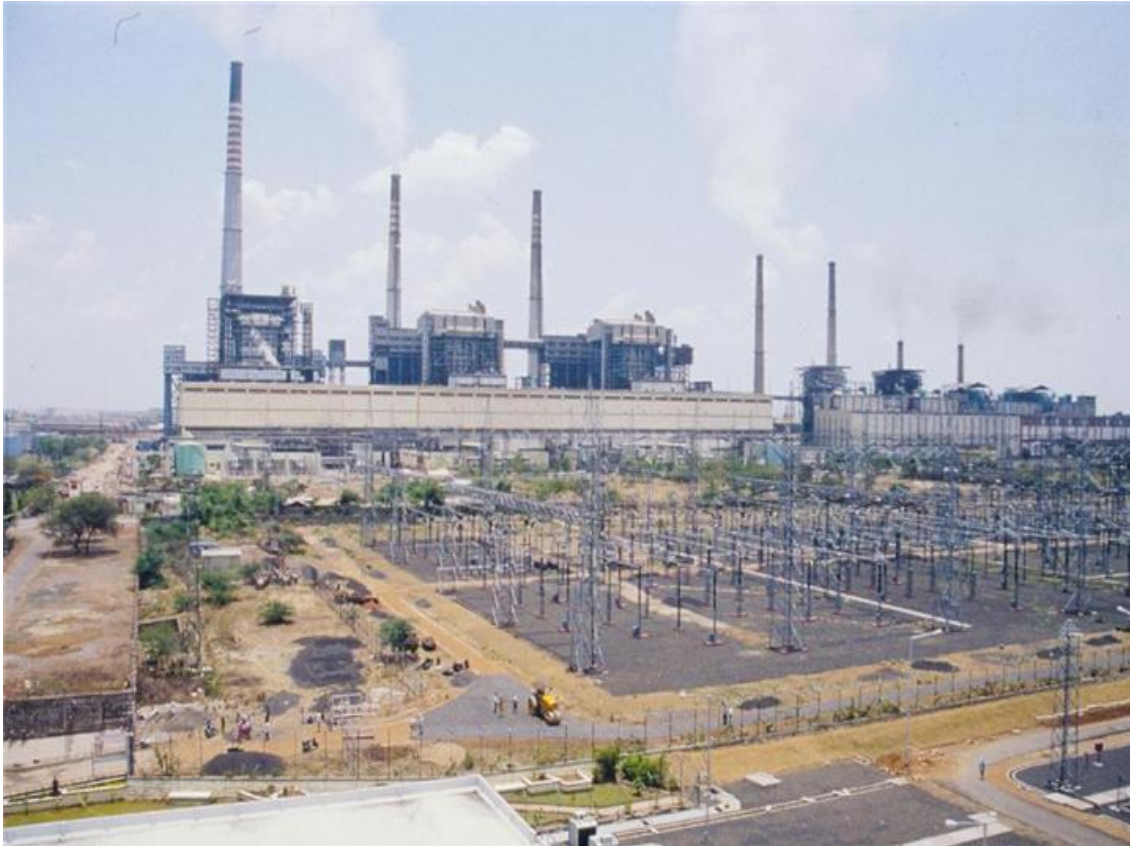
Figure 1.5- Chandrapur-Padghe HVDC Link.
