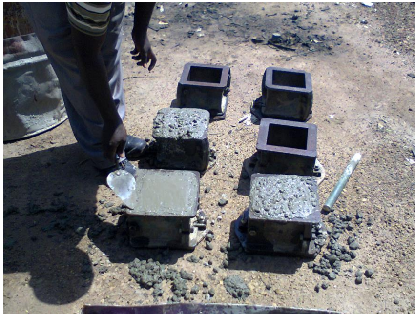
Figure 4.1:-Casting of Cubes
