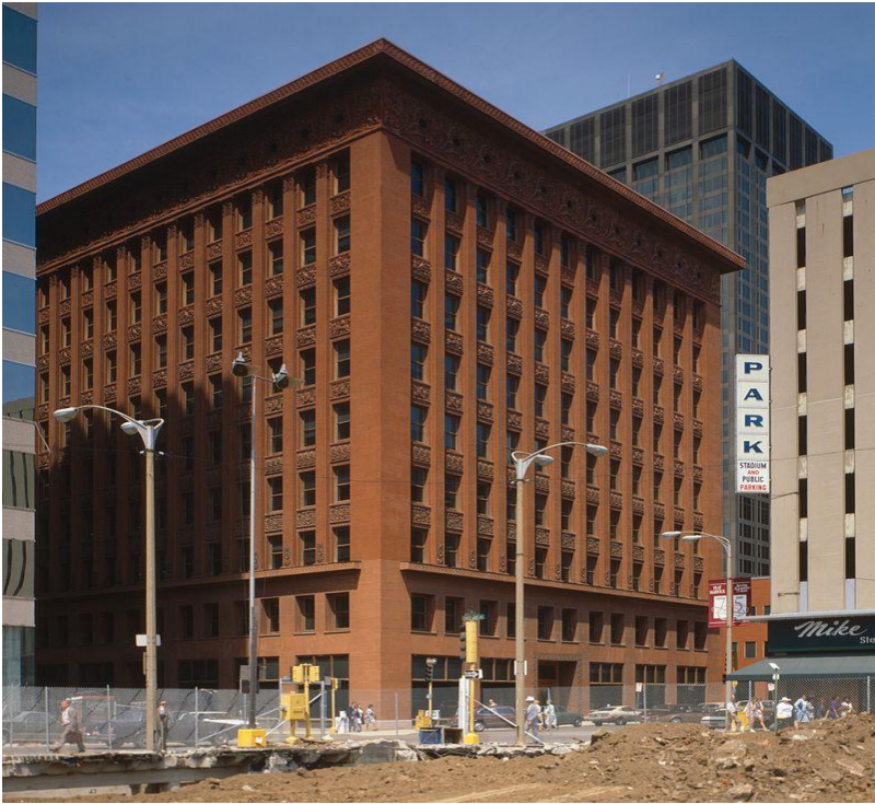
Fig 1.2 The Wainwright Building,10-Storey Building In St. Louis, Missouri, Built In 1891
