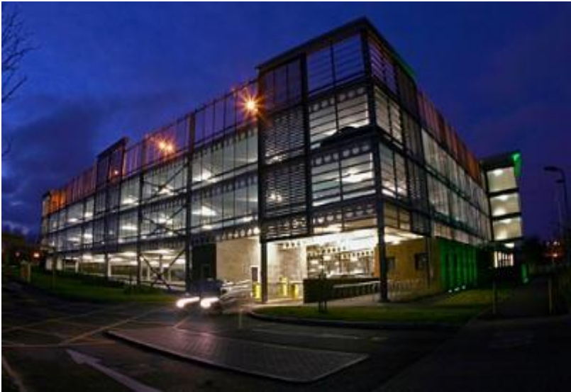
Fig 1.3 Multi-Storey, Steel-Framed Car Park, Milton Keynes in UK
