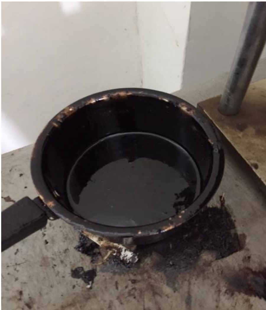
Figure 5.5 heating of bitumen
