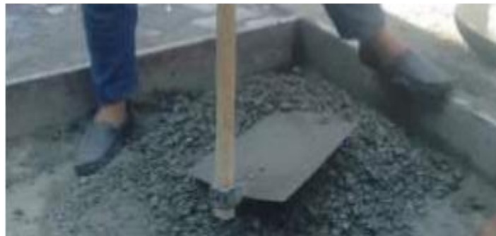
Fig 4.2: Mixing of normal concrete.
