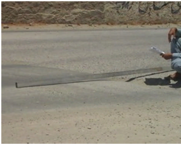
Figure7: High severity Depression
