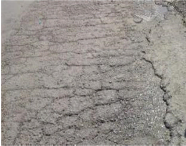
Figure11: Medium Severity Pitching
