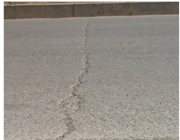
Figure14: Medium Severity Transversers
