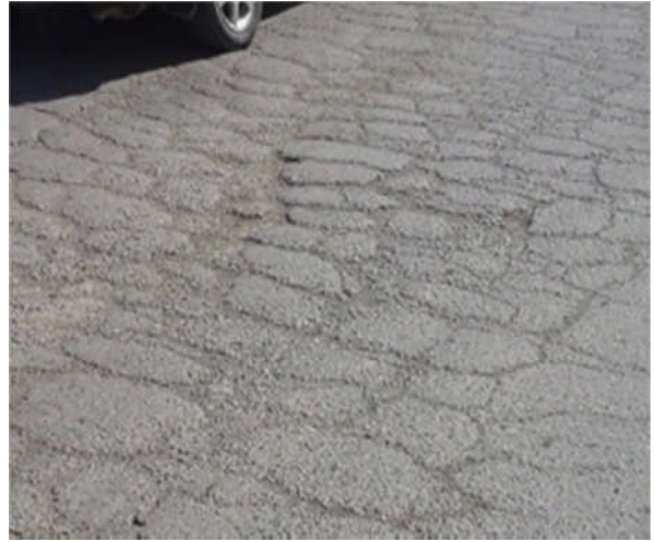
Figure6: Block cracking
