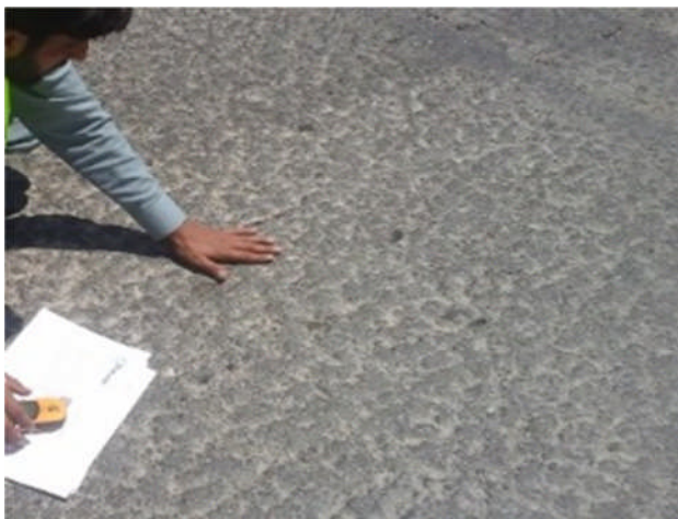
Figure15: Medium Weathering & raveling
