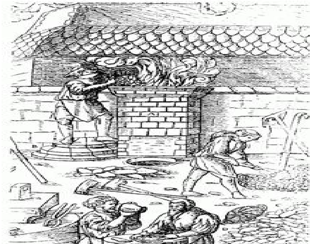
Fig (2) preparation of steel
