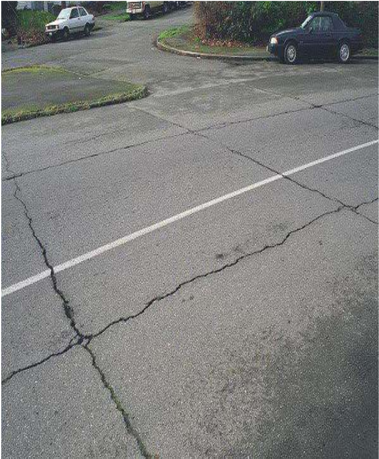
Figure 4-9: Reflection Cracking
