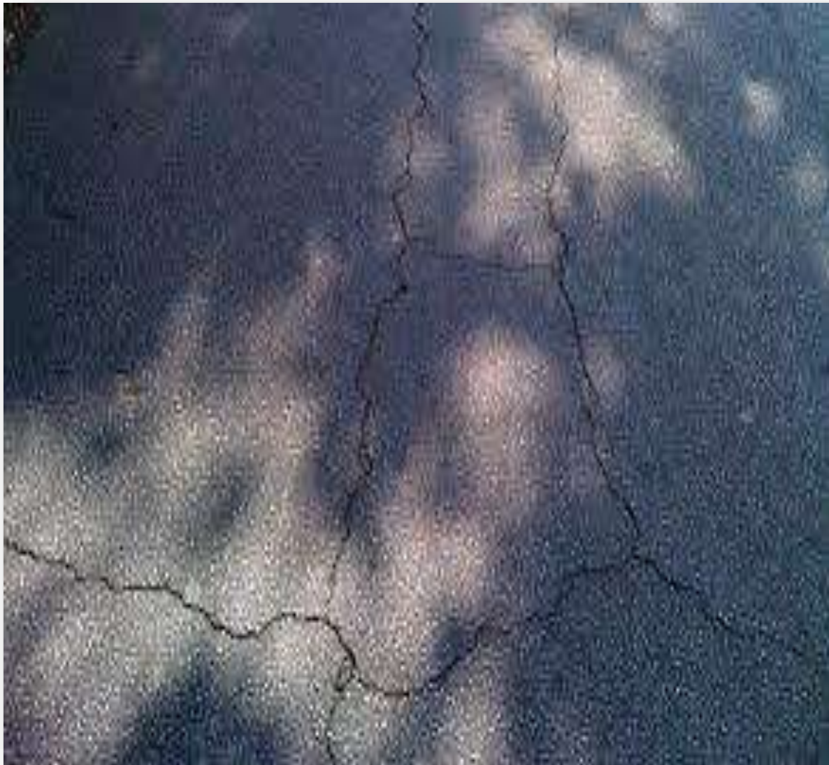
Figure 4-6: Block Cracking
