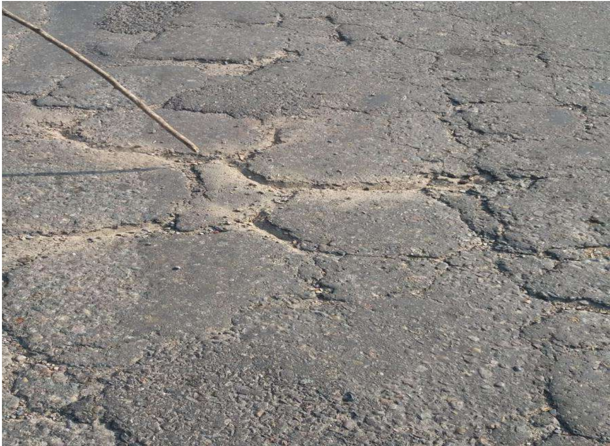
Figure 4-5: Fatigue Cracking
