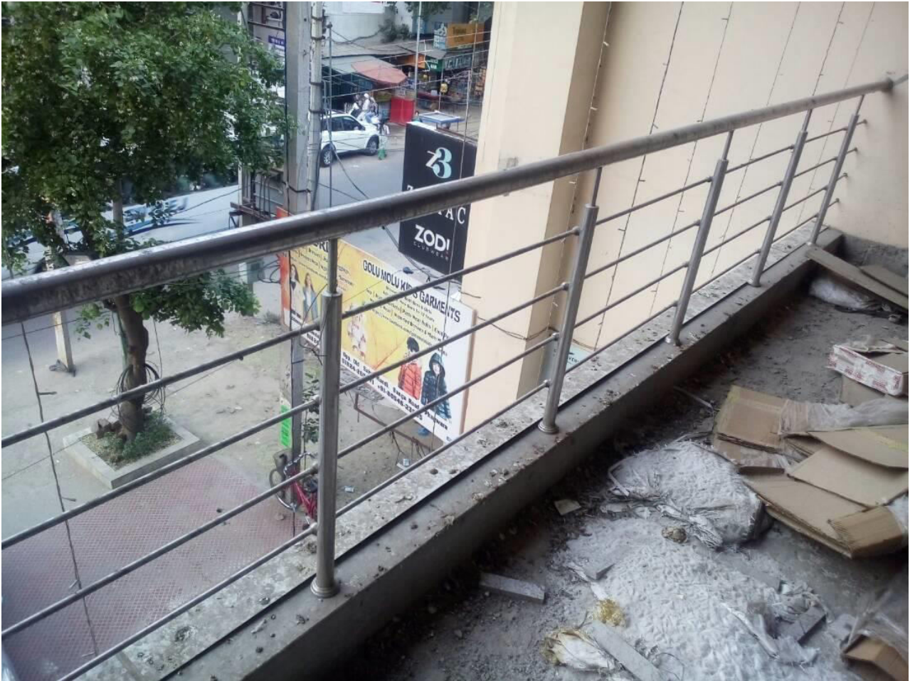
Fig 3.5 Khanduja's third storey (under construction)
