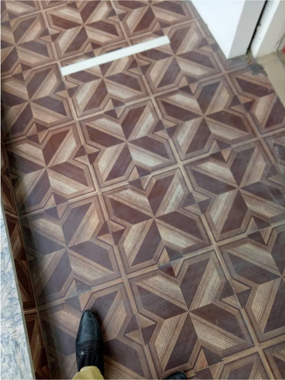
Fig 3.2 View of Floor
