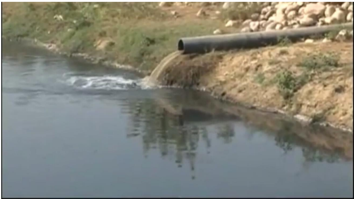
Ropar thermal plant
