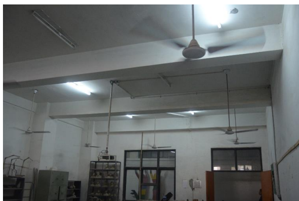
Fig. 22 exposed ceiling of the workshop
