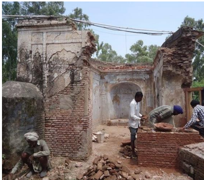
Figure 39: Ongoing Restoration I (authored, 2017)
