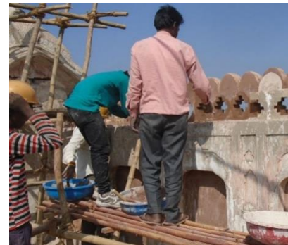
Figure 21: Repair work going on (authored, 2017)
