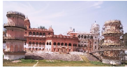
Figure 27: Sheesh Mahal – during restoration (authored, 2017)
