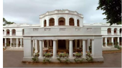
Figure 45: Façade of Palace (Hotel)
