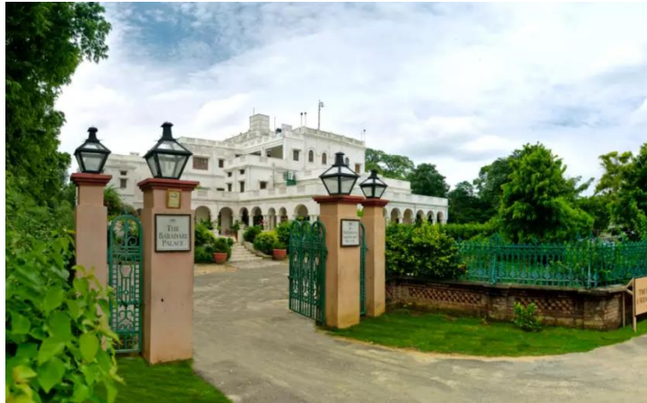
Figure 43: Baradari Palace- Neemrana Hotel entrance (Hotel)
