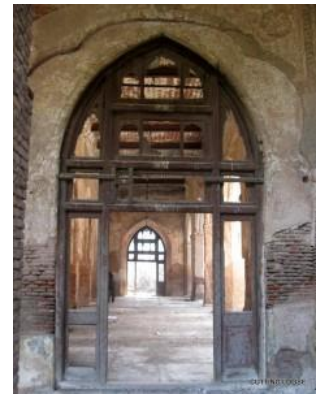
Figure 64: After: Colonial Arch (cutting loose)
