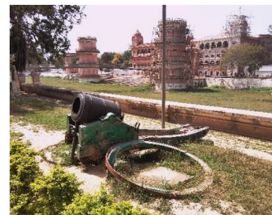
Figure 33: Sheesh Mahal deteriorated view (authored, 2017)
