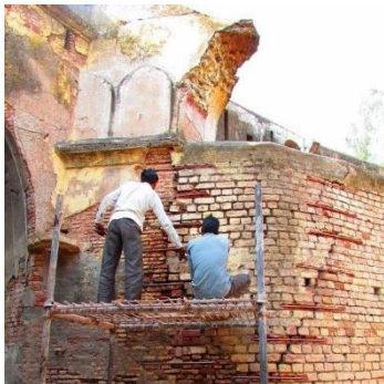
Figure 41: Ongoing Restoration III (authored, 2017)
