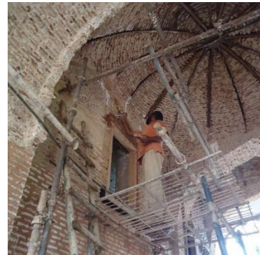
Figure 40: Ongoing Restoration II (authored, 2017)
