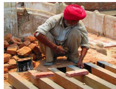
Figure 23: Repair work going on (authored, 2017)
