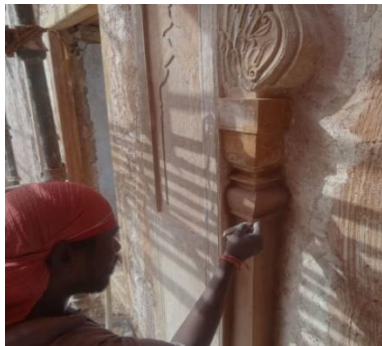
Figure 20: Repair work going on (authored, 2017)
