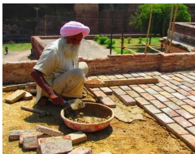
Figure 22: Restore work going on (authored, 2017)
