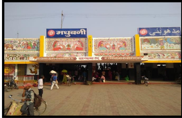
fig no.-18 panting on front façade of railway station.
