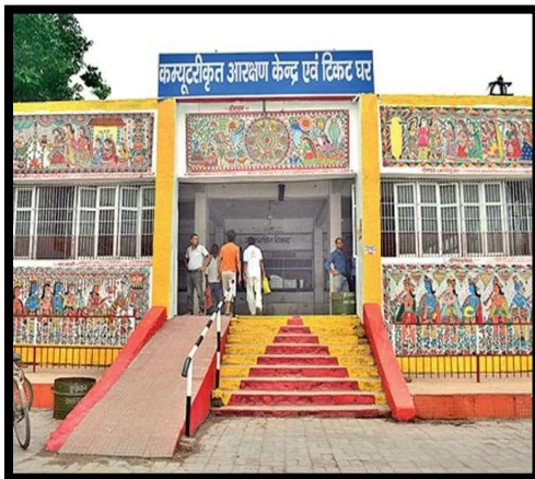
Fig no.21-Painting on outer wall of Reservation center of railway station.
