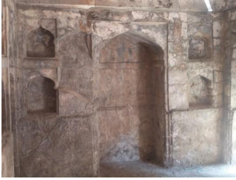
Fig 9. Inside HAMAM (queen's zone)
