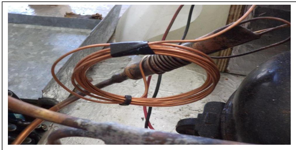
Figure 7.4: Capillary Tube
