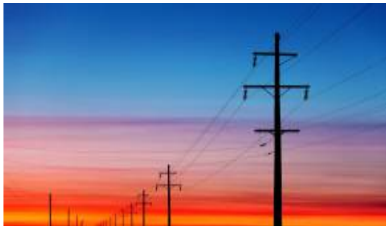
Fig 3.5 Power transmission electrical poles
