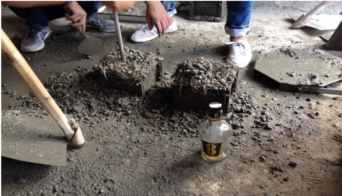
Figure: 6 Moulds prepared (should be left undisturbed)
