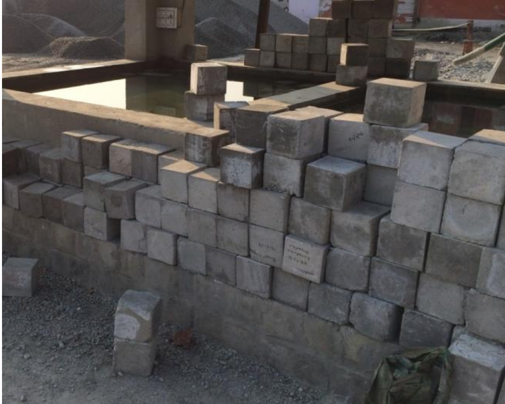
Figure: 7 Cubes taken out from moulds for curing
