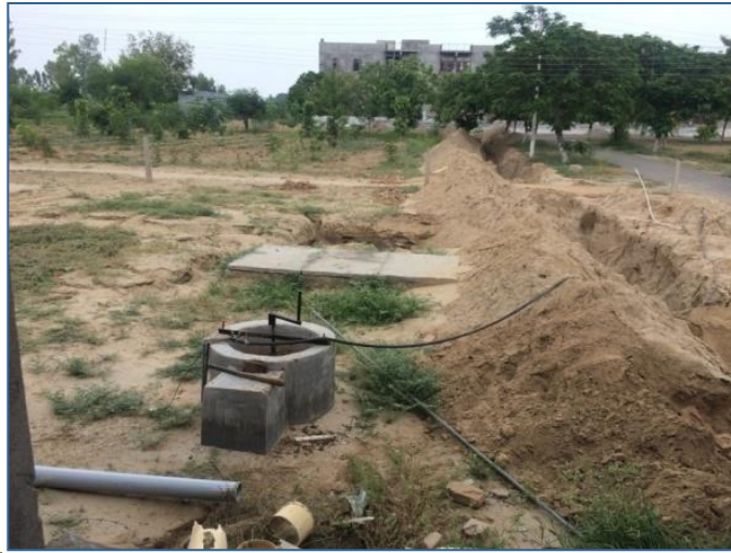
Figure 3.1: Fixed dome biogas plant of capacity 6m 3
