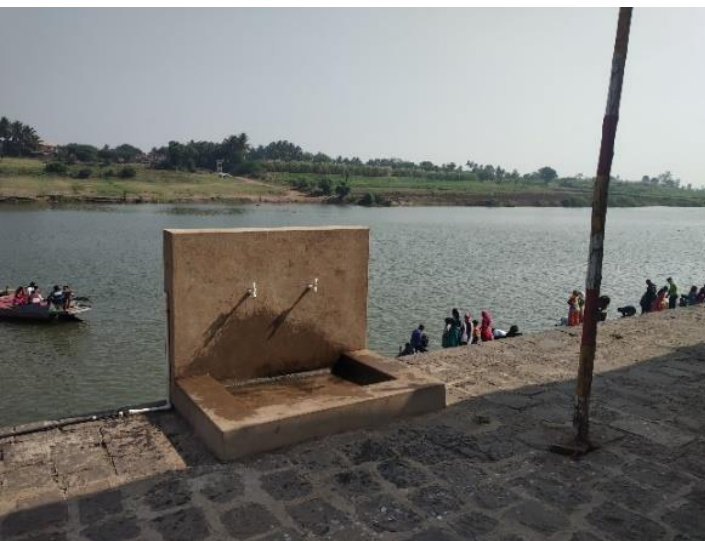
Image 4.30 Provision of drinking water on the upper platform
