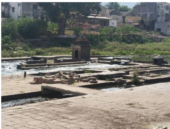
Image 4.13 Water trapped between the broken steps of ghats,
