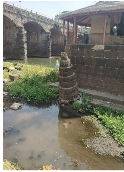
Image 4.12 Loose stones are lying around on the platforms of Brahmanshahi ghats, Wai
