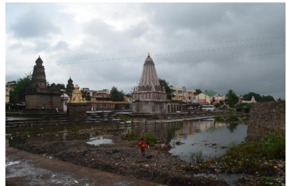
Image 4.2 Causeway connecting Ganpati ghats and another bank of Krishna River Source: Photographs taken by the scholar on-site
