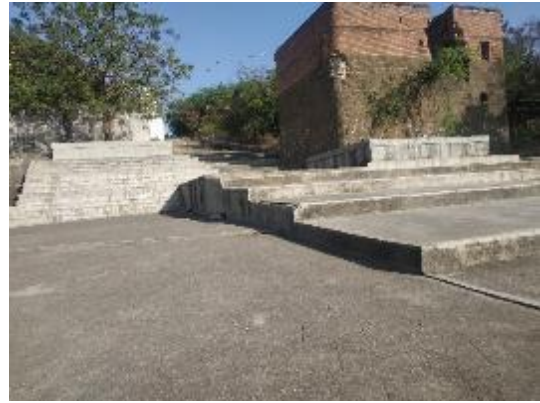
Image 4.60 Clean and repaired structures of Naag
