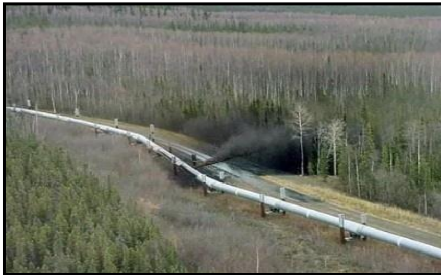
Figure 1.5 Oil spills due to Pipeline failure [6]
