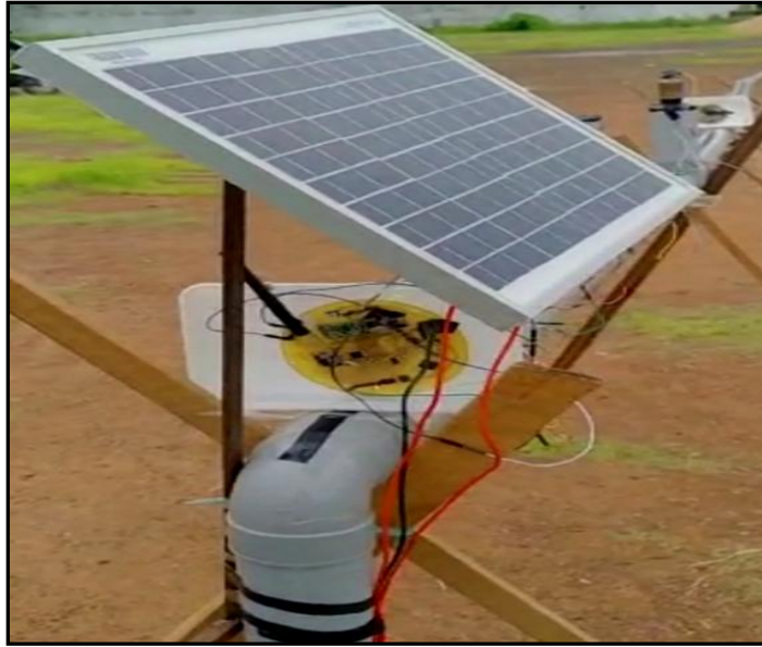
Figure 7.1 Sensor node with solar on the pipeline
