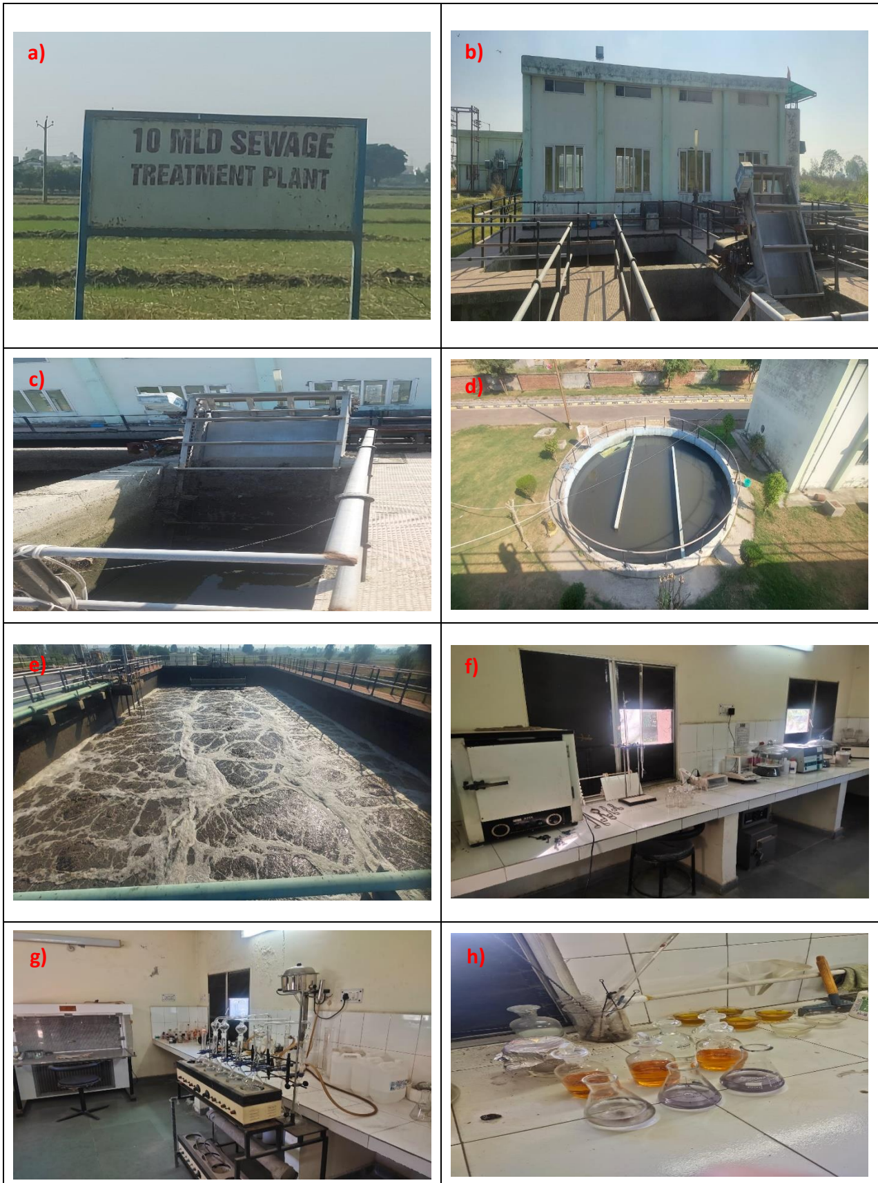
Figure 3.5. 10 MLD Sewage treatment plant, a) STP capacity, b) Automatic screens, c) Fine screens, d) Processed wastewater chamber, e) Aeration chamber, f) Lab set-up, g) STP lab, h) Testing equipment's
