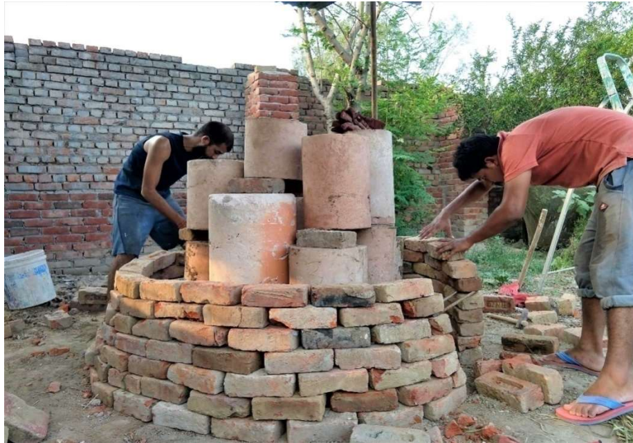
Figure 3.4.9 Sculptors creating local dewaxing kiln with terracotta bricks
