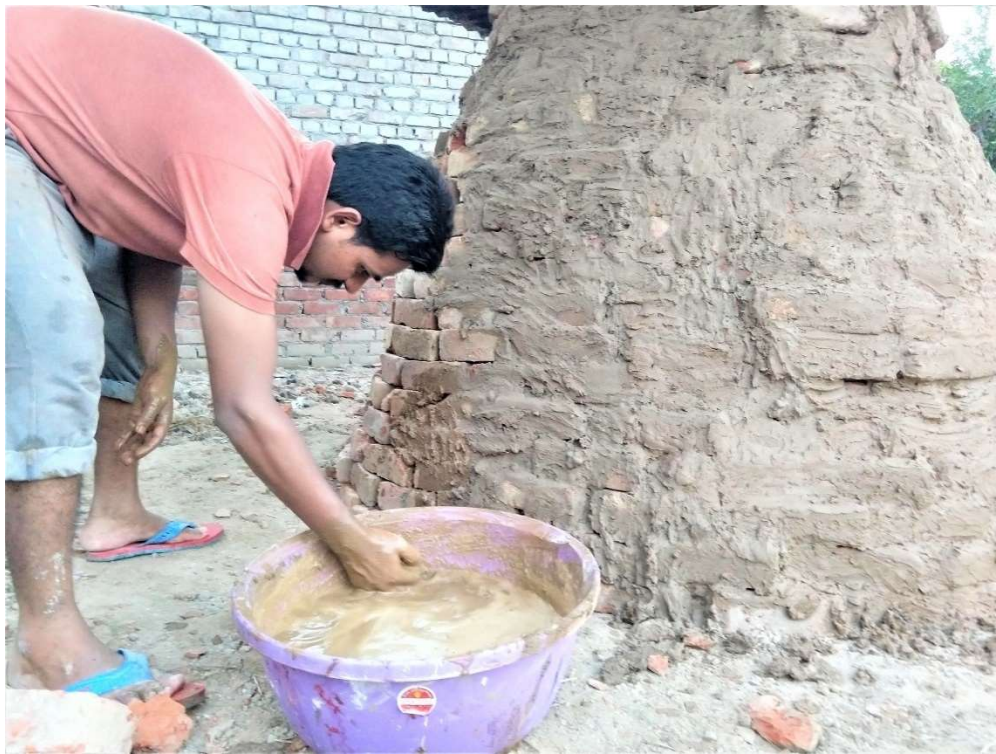
Figure 3.4.10 Sculpture applying clay slip to seal the bricks gap of local kiln
