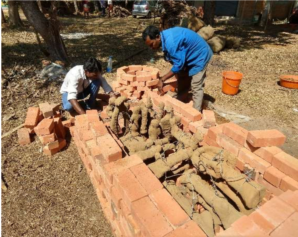
Figure 3.2.16 Local kilns is prepared with bricks
