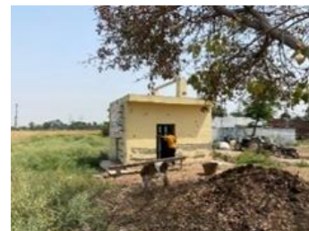
Fig. 4.26 Faulty supply pump
