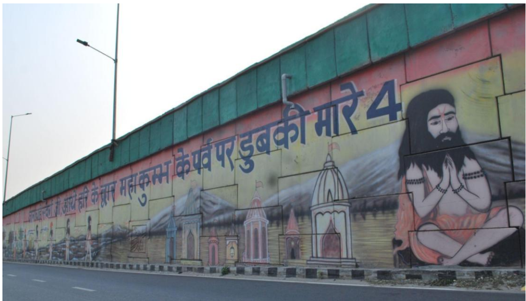
Figure 4.2.2.1.66 and 4.2.2.1.67. Pipli chowk Bus Stand , Grand Trunk Road, Pipli, Kurukshetra, Haryana, Self Clicked
