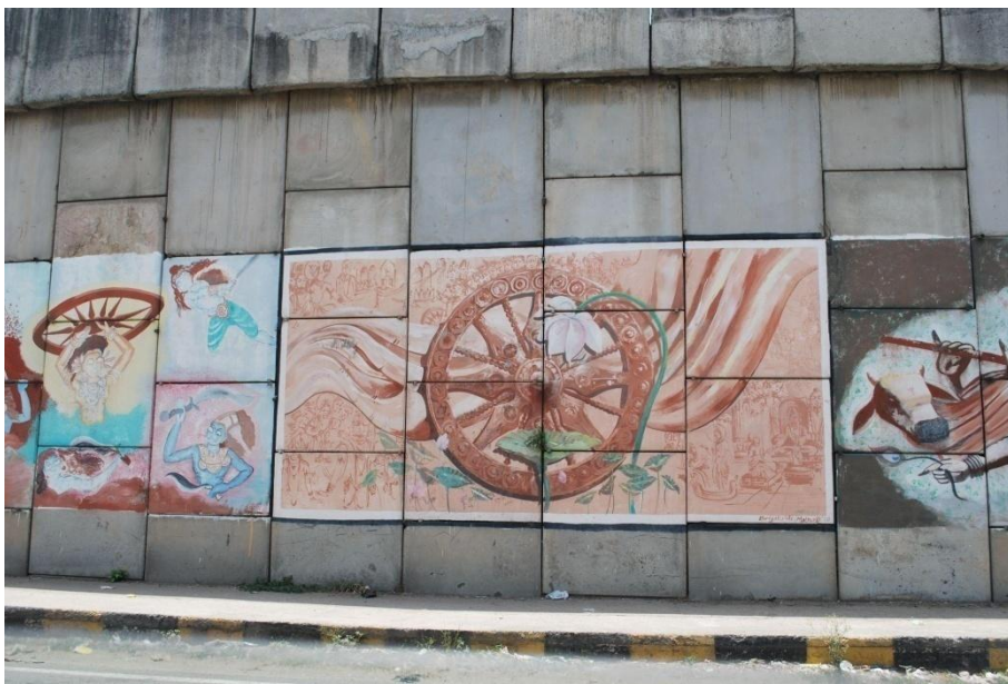
Figure 4.2.2.1.51 and 4.2.2.1.52. Pipli chowk Bus Stand , Grand Trunk Road, Pipli, Kurukshetra, Haryana, Self Clicked
