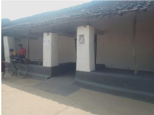
Fig. 230: Raised Platform at the Entrance
