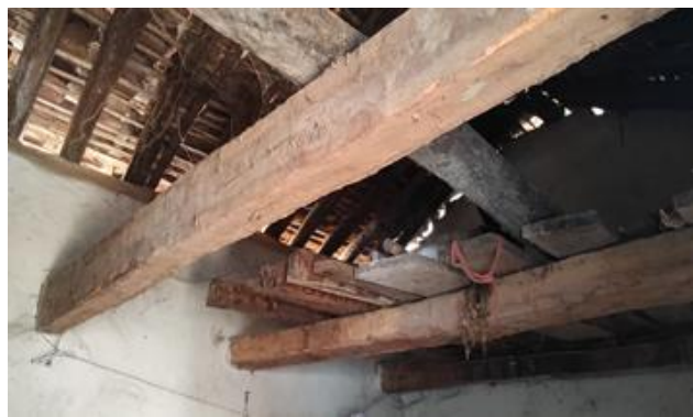
Fig. 268: Post Supporting Roof
