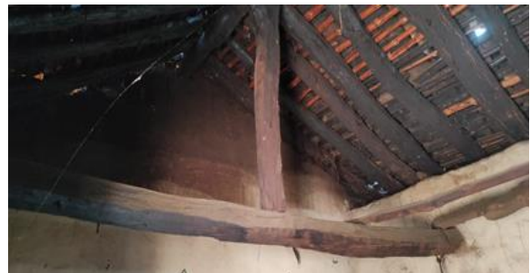
Fig. 270: King Post in Sloping Roof
