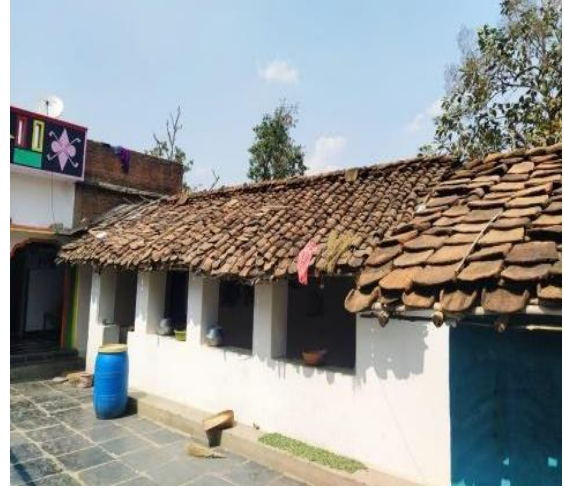
Fig. 195: Adjoining Old Structure of Dwelling Unit
