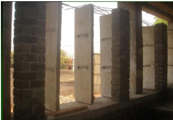
Fig. 117: Window Fins during Construction
