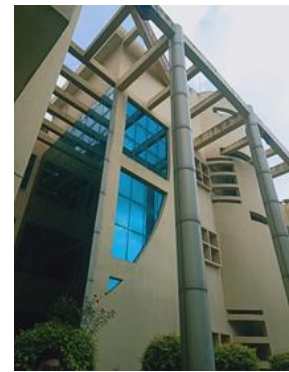
Fig. 112: External Shading
