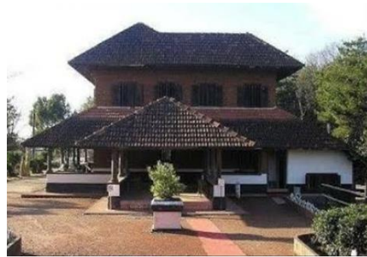
Fig. 25: View of Entrance
