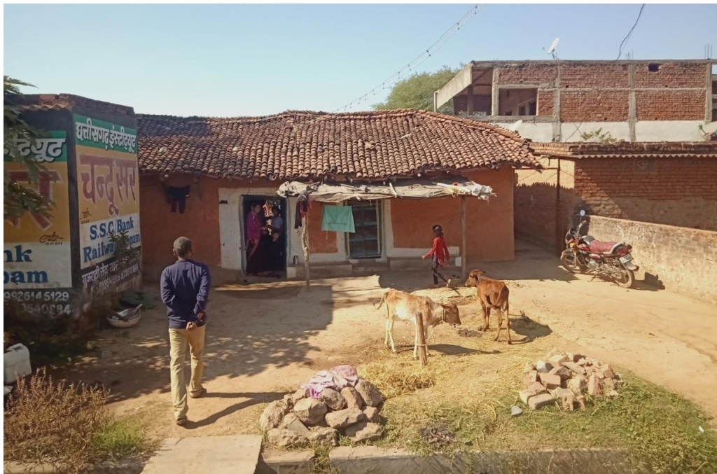
Fig. 140: Front View of Dwelling Unit at Borsi, Chhattisgarh
