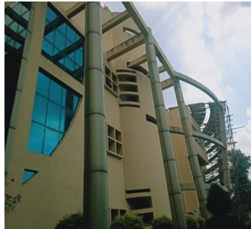
Fig. 98: View from Northwest
