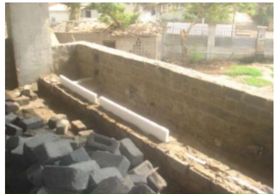
Fig. 120: Thermal Insulation in Wall
