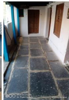
Fig. 132: Slate Flooring at Passage
