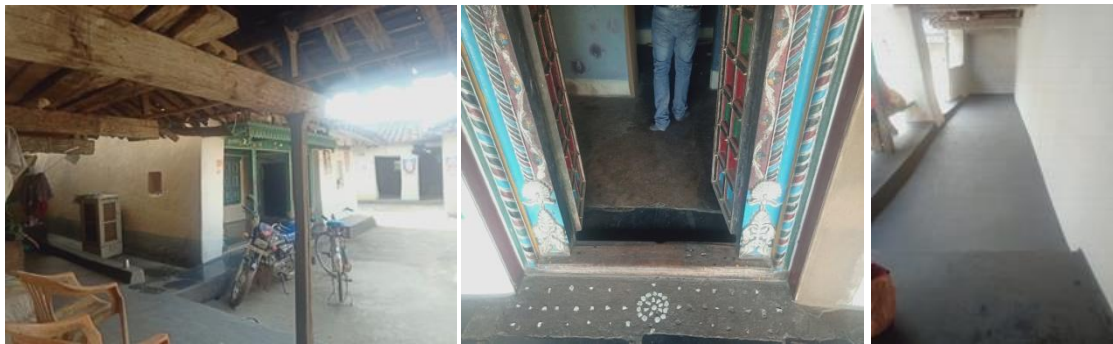
Fig. 242: Timber Post Supporting Overhangs Fig. 243: Door Frame Fig. 244: Tyre Flooring
