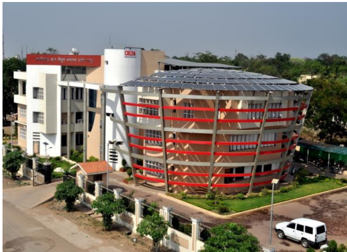
Fig. 99: View from Southwest
