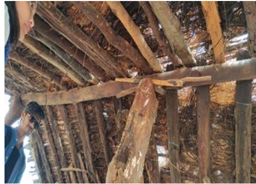
Fig. 272: Ridge Supported by Timber Post
