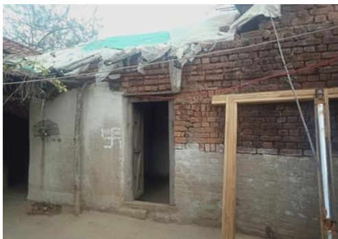
Fig. 221: 15" Th. Brick Wall with Cement Plaster
