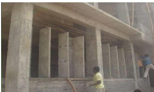
Fig. 121: Egg Crate Devices during Construction
