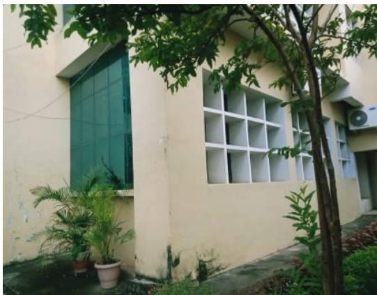
Fig. 108: Egg Crate Shading Device
