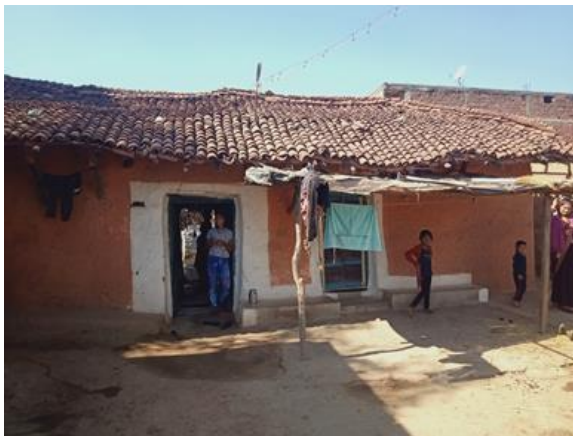
Fig. 143: Raised Platform at the Entrance
