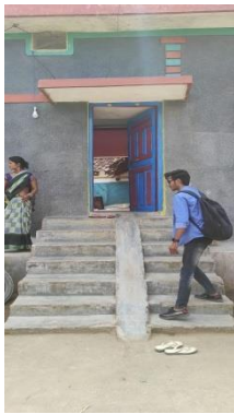
Fig. 266: Steps and Ramp at the Entrance
