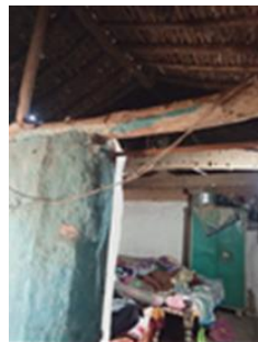
Fig. 151: Timber Trusses in Roof
