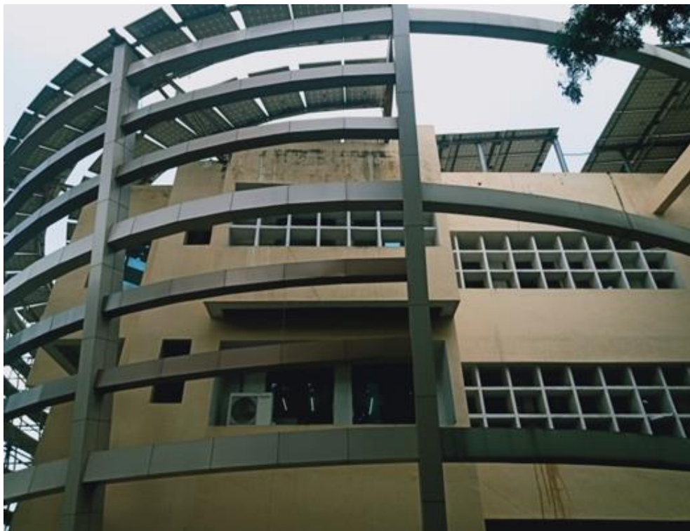
Fig. 107: Southwest Umbrella as Shading Device
