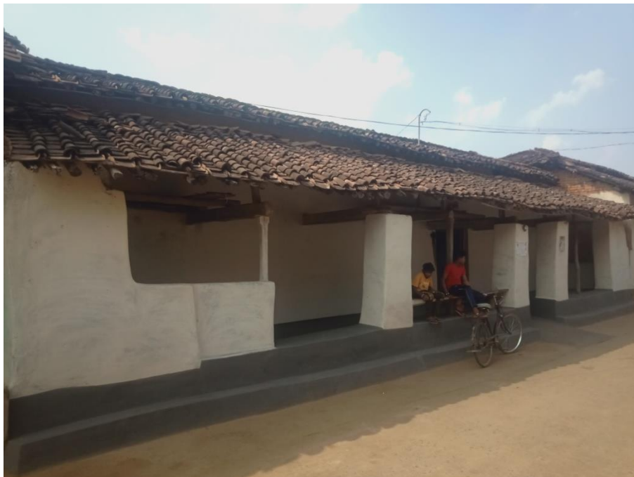
Fig. 227: Front View of Dwelling Unit at Mohradih, Chhattisgarh
