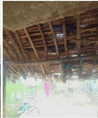
Fig. 199: Roof Supported by Battens & Purlins
