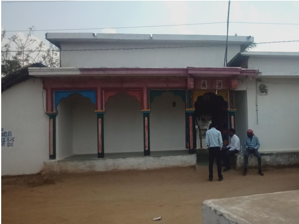
Fig. 167: Front View of North-Facing Dwelling Unit at Chhattarpur, Chhattisgarh
