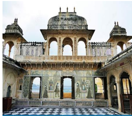
Fig. 49: Part of Domical Roof Is Always Shaded (Source: Pinterest, n.d.)
