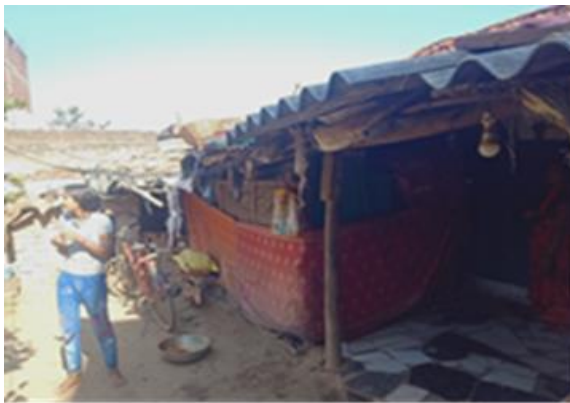
Fig. 148: Kitchen Walls Covered with Cloth
