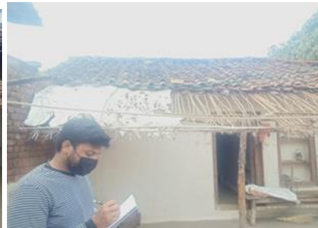
Fig. 219: Sloping Roof Supported by Wooden Post
