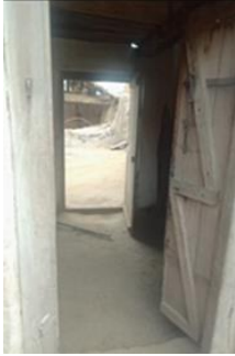
Fig. 224: Passage towards South
