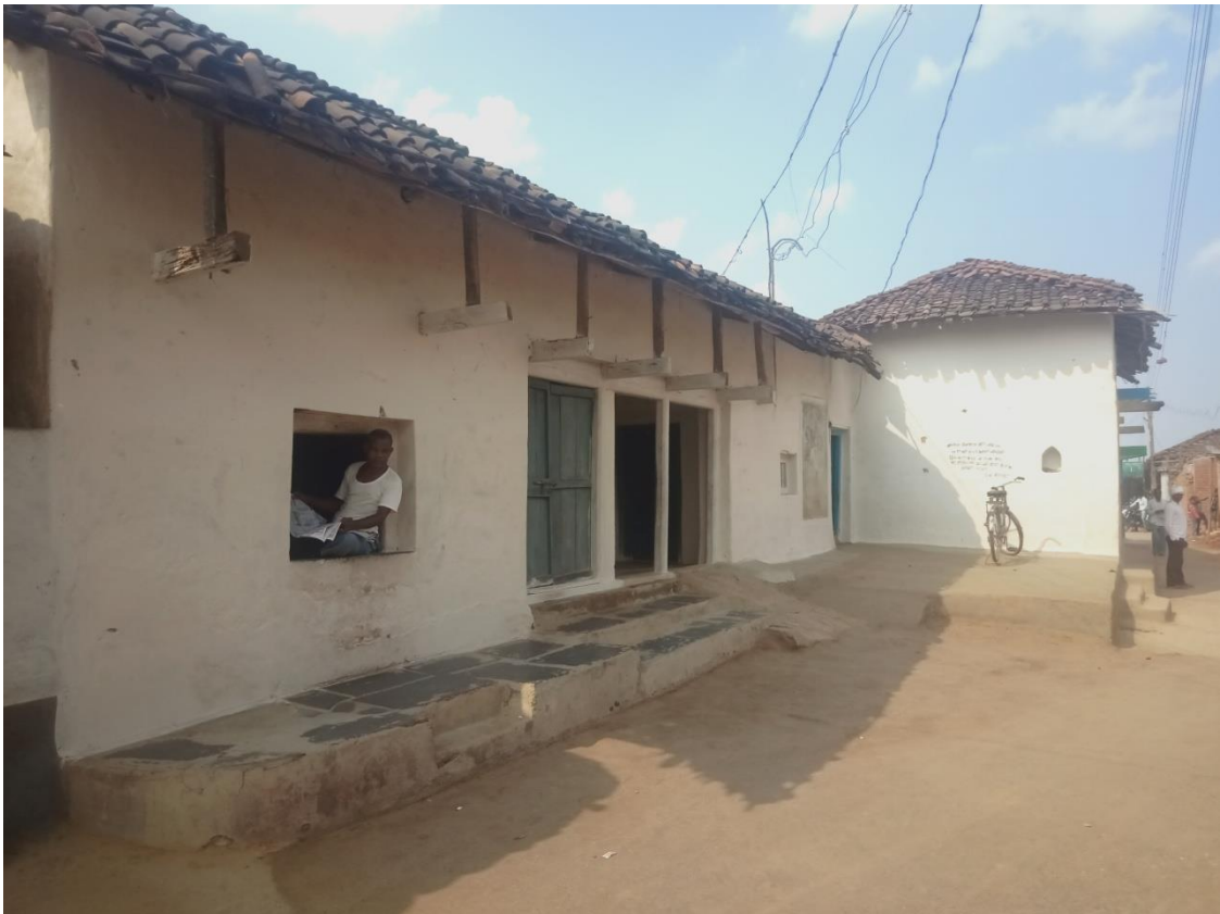
Fig. 245: Front View of Dwelling Unit at Mohradih, Chhattisgarh
