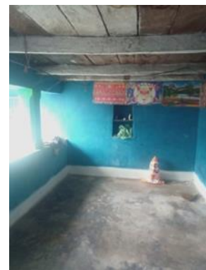
Fig. 189: Lobby with Cement Flooring and Timber Roof
