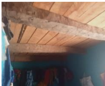
Fig. 211: Timber Roof Supported by Purlins
