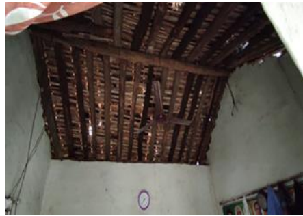
Fig. 225: View of Roof from Inside
