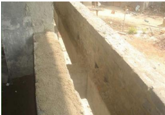
Fig. 119: Permanent Shading Device in the Form of RCC Pergola
