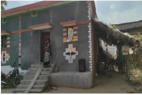
Fig. 264: View of Dwelling Unit from Southeast
