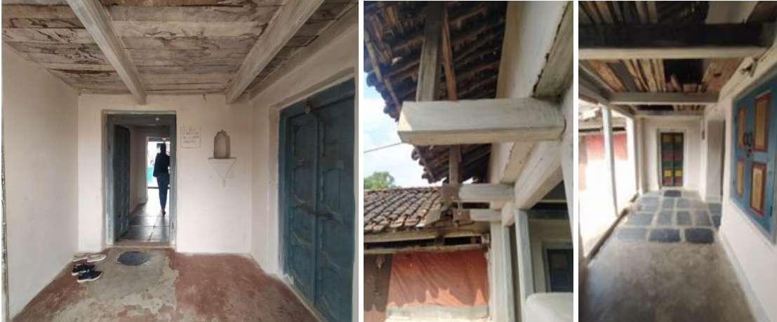
Fig. 250: Lobby at Entrance Fig. 251: Post Supporting Roof Fig. 252: Passage
