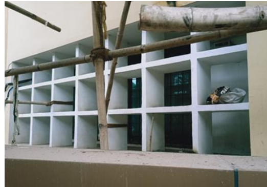
Fig. 116: Egg Crate Shading Device
