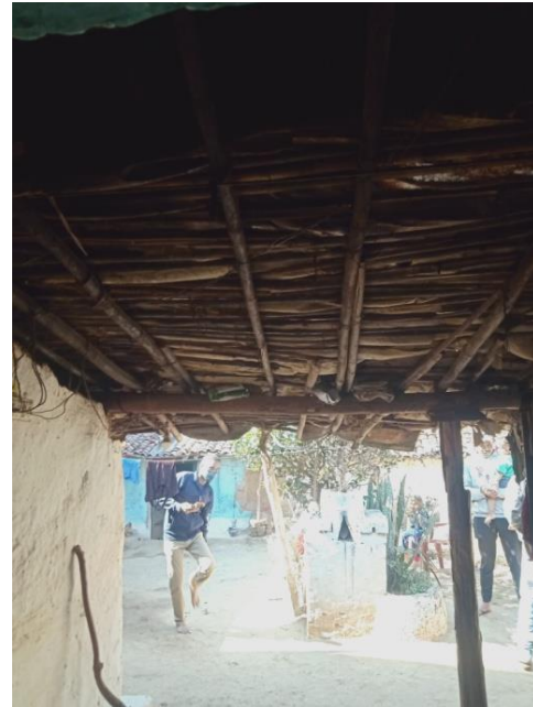
Fig. 142: Timber Roof Supported by Wooden Post
