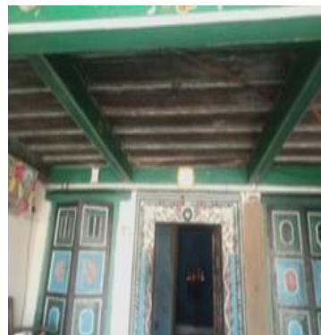
Fig. 237: View of Kitchen Roof
