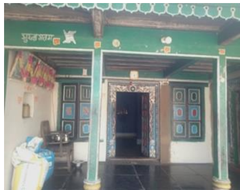
Fig. 236: Front View of Kitchen at South
