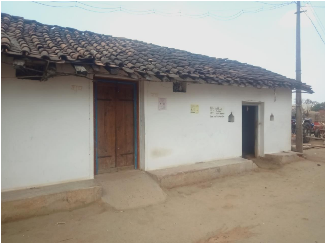
Fig. 82: Rear Facade of Dwelling at Village Dagania, Distt. – Durg
