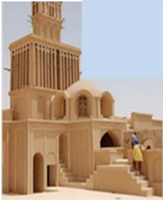
Fig. 71: Wind Tower in Jodhpur Hostel to Catch Favourable Cool Wind from Southwest for Passive Cooling
