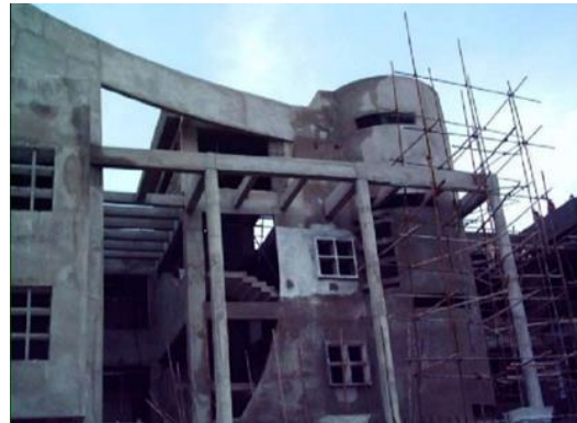
Fig. 118: West Elevation during Construction
