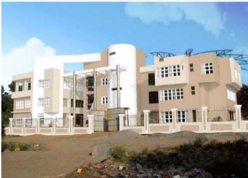
Fig. 106: Front View from West during Construction
