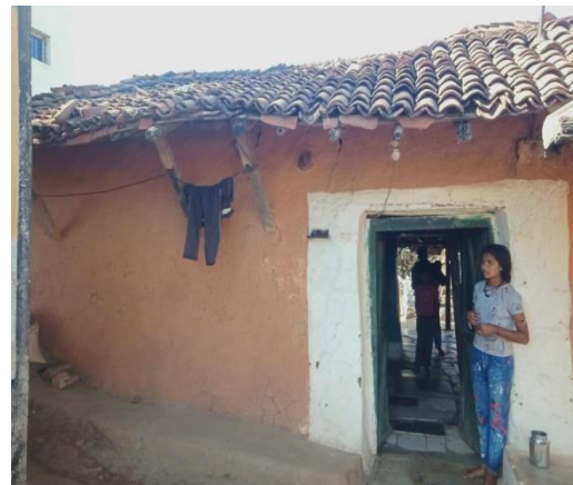
Fig. 144: Entrance Door Highlighted with Lime Wash
