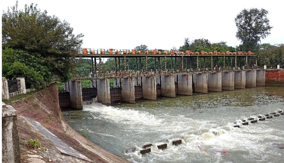
Plate 2.9: Installation of water management gates to regulate the water flow at Kanjli Wetland
