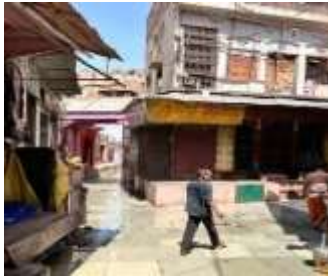
Figure 3.35 13 zone 3-existing condition at Vishram ghat
