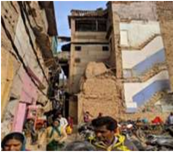
Figure 5.9: Large Scale Demolition of Local's Houses and unjustified compensation and poor rehab situation
