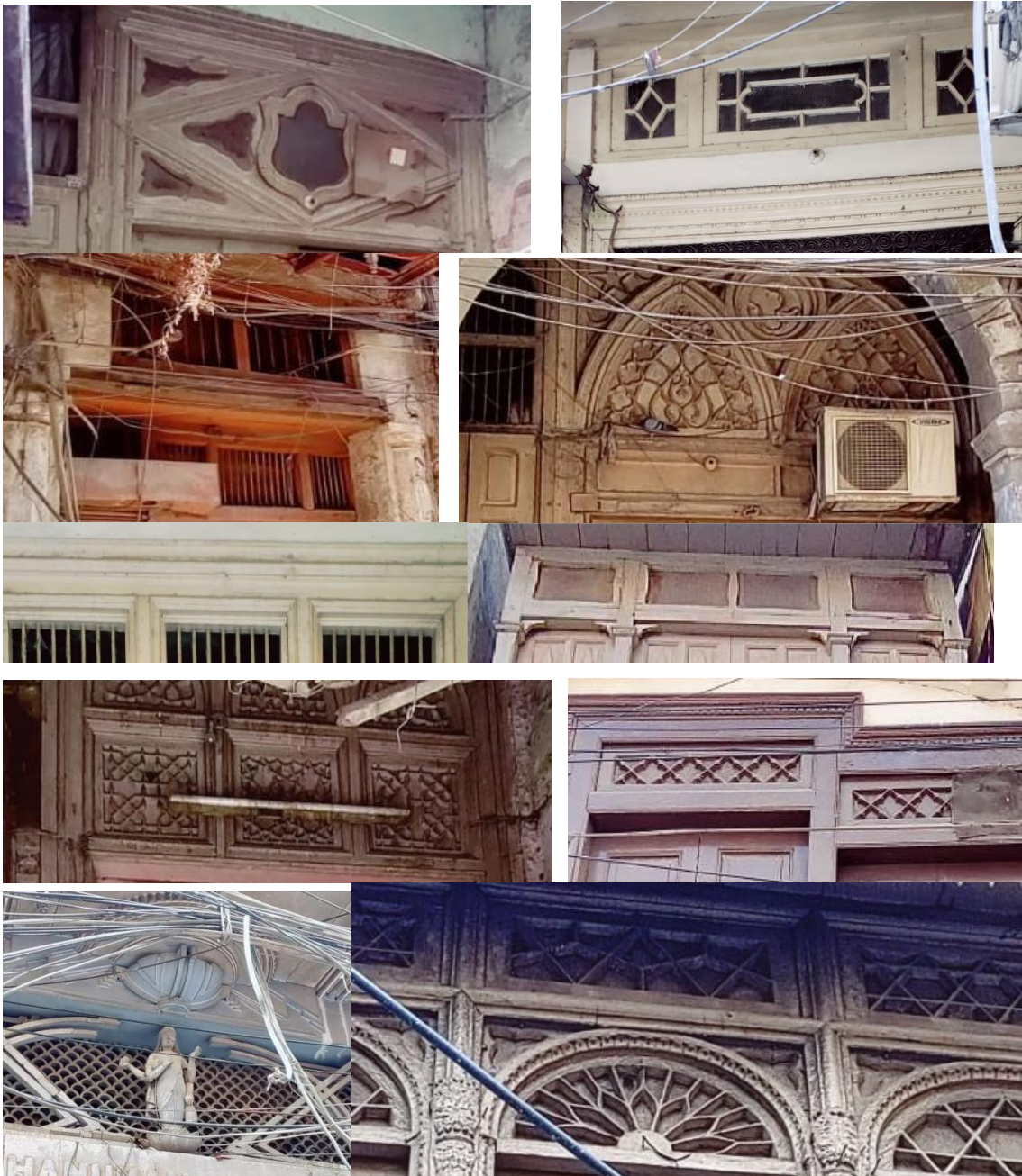
Figure 5.9: Images showing Wooden work on Doors and window (Transom)
