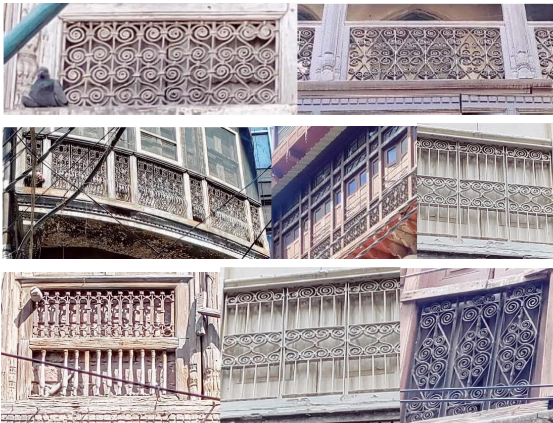
Figure 5.15: Various types of M. S. Grills in Katra Ahluwalia
