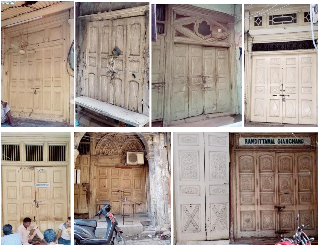
Figure 5.7: Images showing Panelled doors with arch character/ventilators
