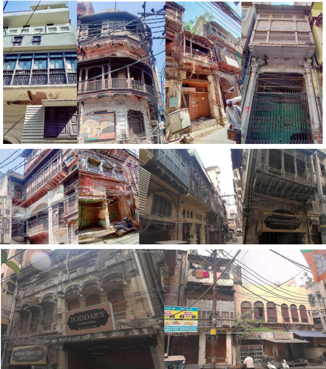
Figure 5.1: Present situation of structures of Katra Ahluwalia.
