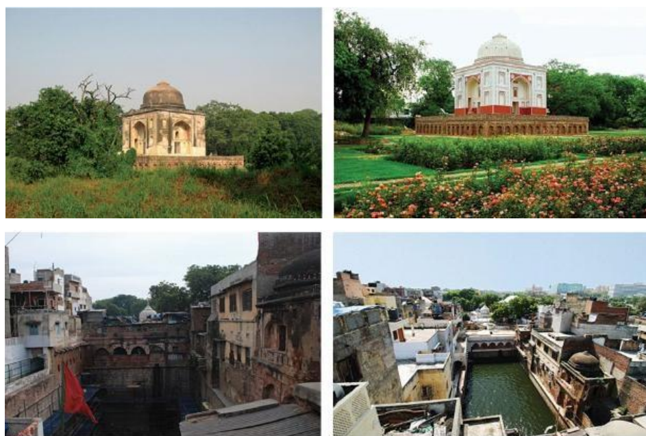
Figure 2.6 : Lakkarwala Burj and Nizamuddin Baoli: before & after conservation
