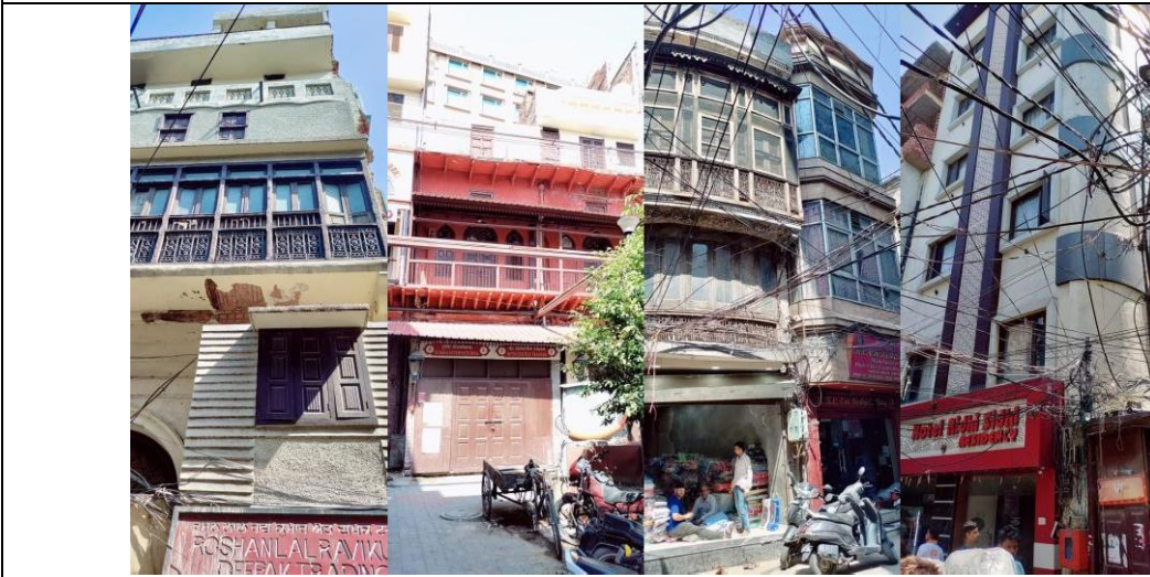
Figure 4.16: Modern Developments In Katra Ahluwalia
