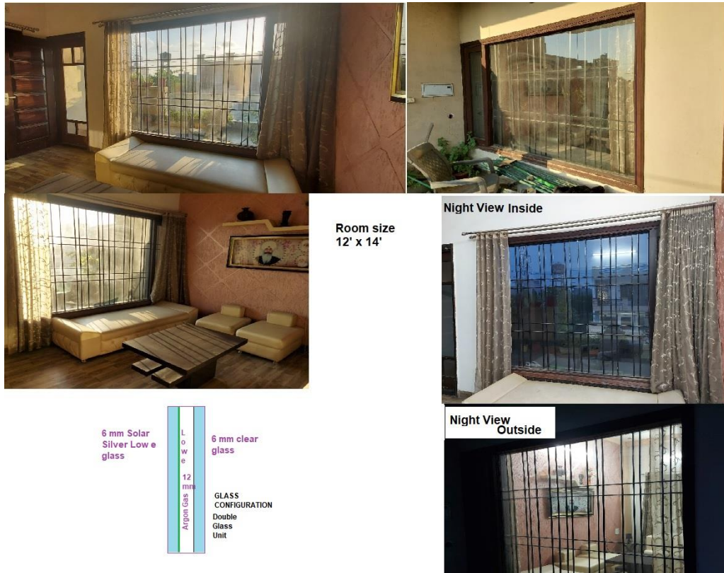
Figure 4.9 The view of room for the installed DG3 fenestration
