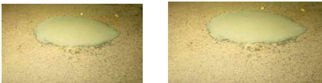
(a) CC Pot Hole filled with SCC HyFR-NA1.0 (b) Pot Hole filled with SCC HyFR-NA1.5 Fig.6.12 Pot Holes repaired with two types of fast-setting SCC HyFR-NA recipes
