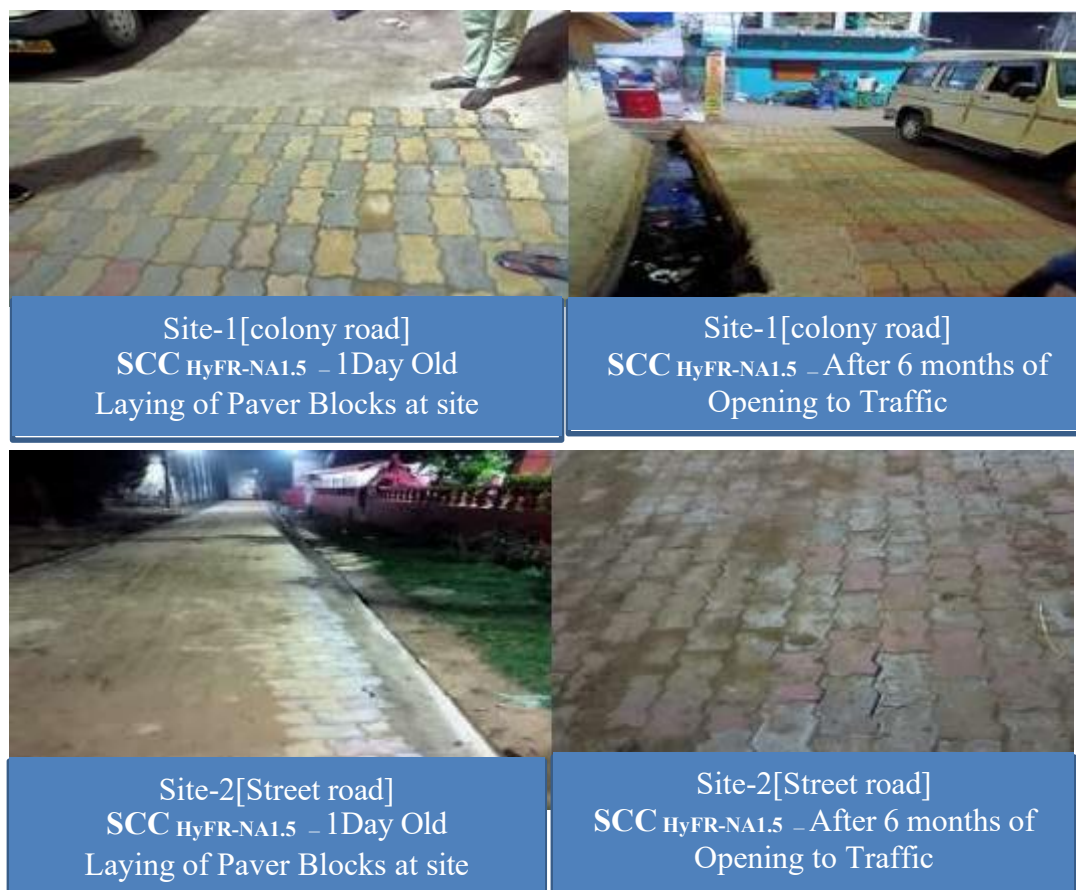
Fig. 6.17 View of Precast Paver Block Pavement trials carried with SCC HyFR-NA1.5
