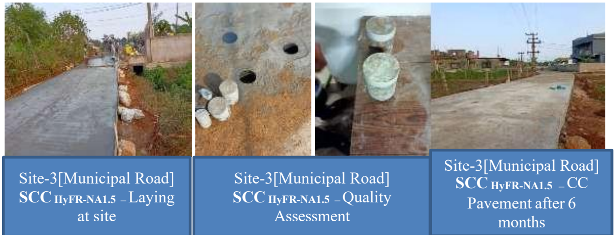
Fig. 6.18 View of CC Pavement site- trials carried with SCC HyFR-NA1.5
