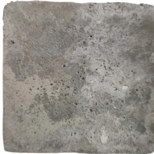
Figure 54: ECC Cube after Chloride Attack
