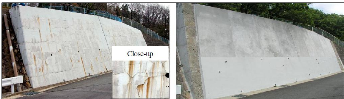
(a) Before repair
