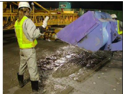
(c) Placement of HSPFRCC
