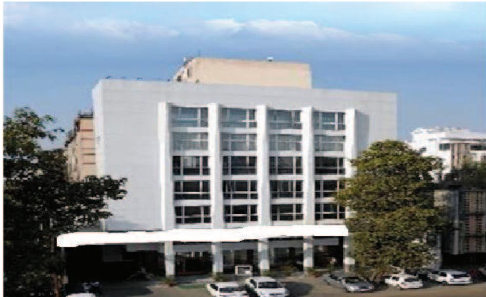
Figure 3.2: Building used in the case study (site photograph)
